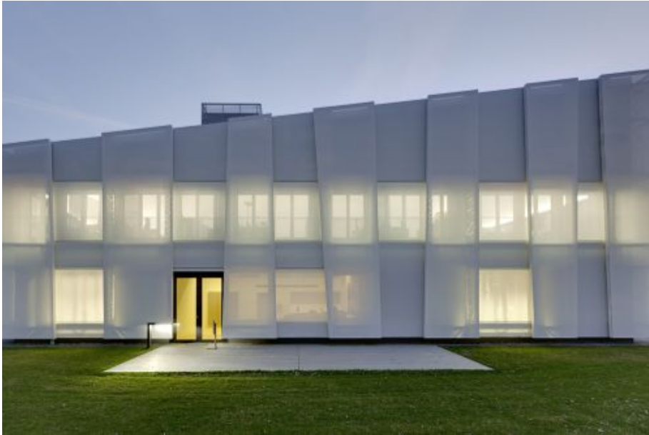
Figure 1.7: R&D center in Dogern, Switzerland, 2010 (from www.detail-online.com ).
