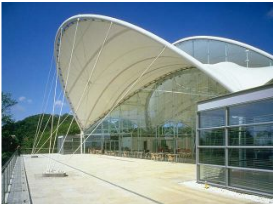
Figure 1.1: SAGA Headquarters Amenity Building, Folkston, UK, 2002 (from www.skyspan.com ).
