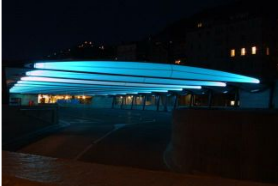
Figure 1.6: Garage Park in Montreux, Switzerland, 2004, realised with Tensairy beams (from www.canobbio.com ).
