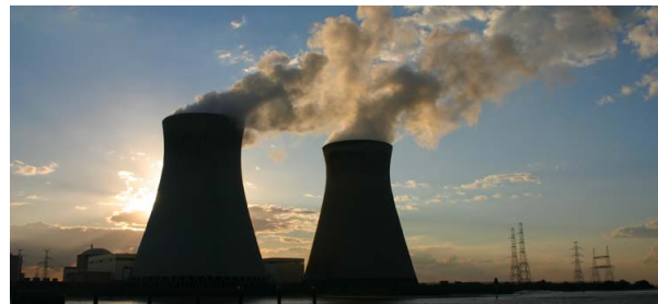
(c) Chimneys in a nuclear powerplant.
