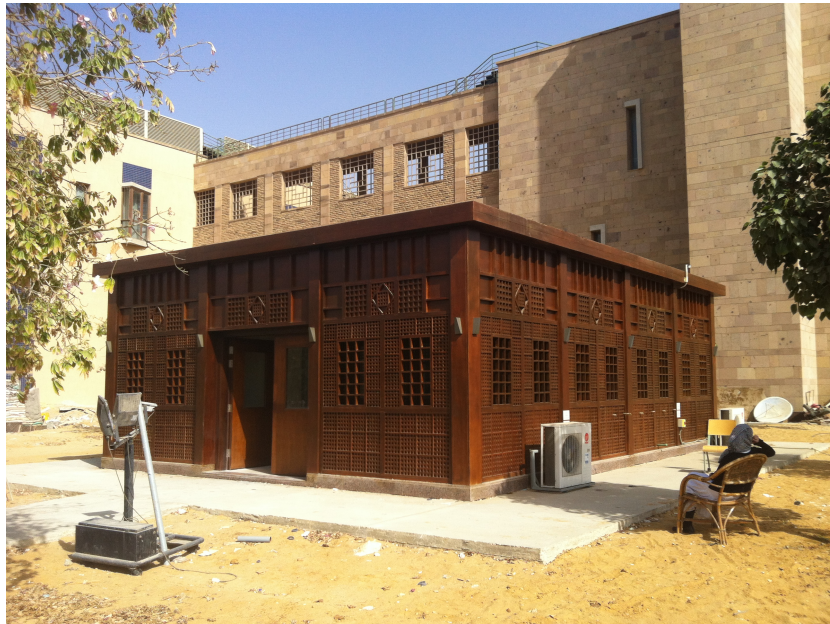
Figure 4.2: South-west view of the desalination laboratory
