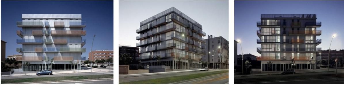
Fig.6.2.1. (Left/ Middle/Right) Transformation of the facade of the building. Picture source: [http://www.narch.eu/p7/p7.html (accessed 15 th February 2014)]
