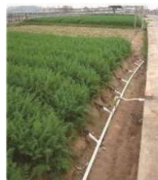
FIGURE 10 LOW-PRESSURE CANAL PIPE
