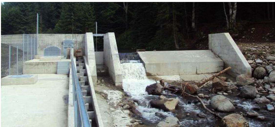
fig. 3 - View of the Hålmätgel tyrolean type intake with sluice gate, fish ladder and covered silt basin.
