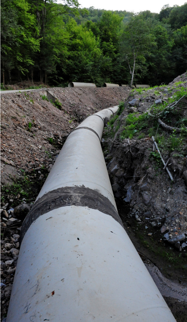
fig. 5 - View of the Rapid Pipeline before covering
