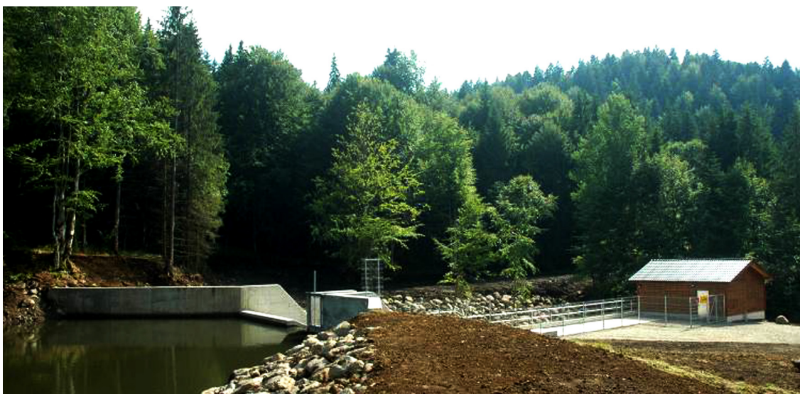
fig. 4 - View of the Hålmätgel small accumulation basin surrounded by artificial reinforced concrete walls and stone walls, and upstream control house.
