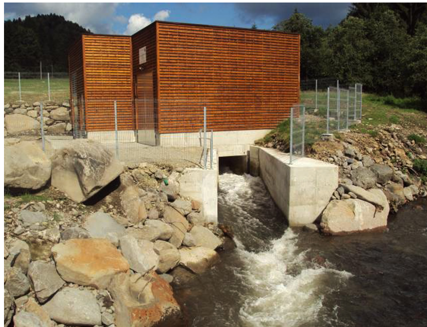
fig. 7 - View of the Hălmăgel Powerhouse and the tailrace, with the water that was turbined, flowing back to the Hălmăgel river.
