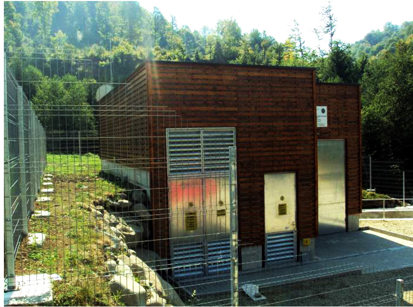
fig. 6 - View of the Hălmăgel Powerhouse
