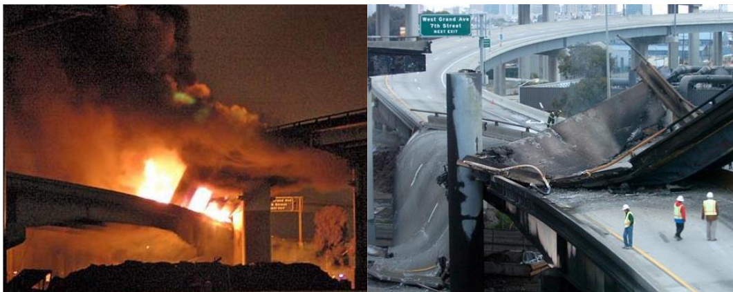
Fig.1. 9 McArthur Maze Collapse by Fire
