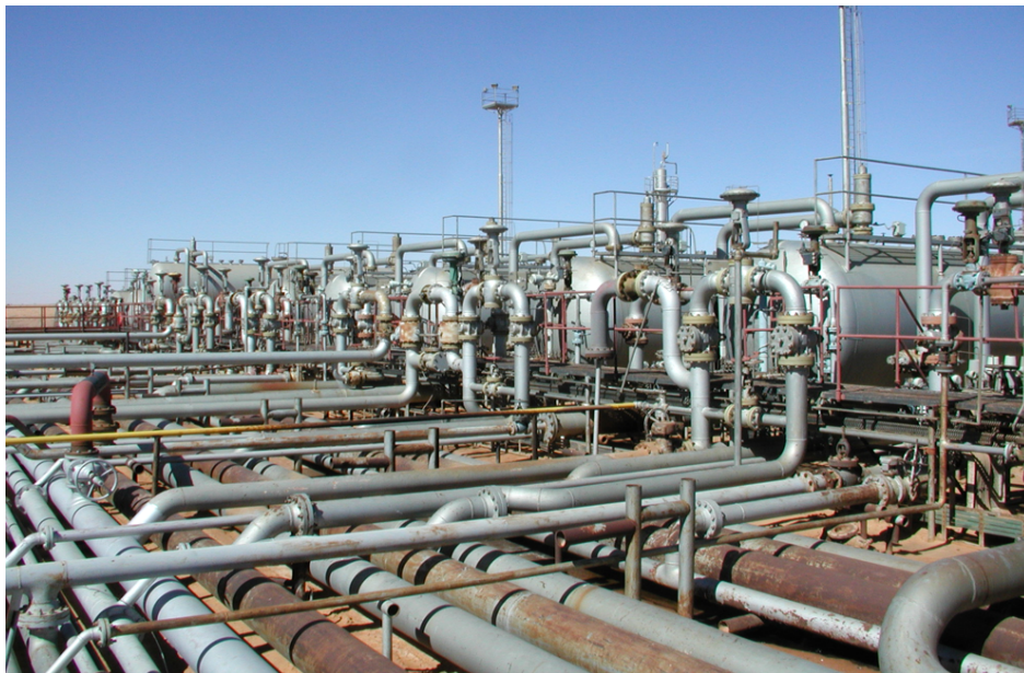
Figure 1.1: Three-phase separators in Trecate oil field
