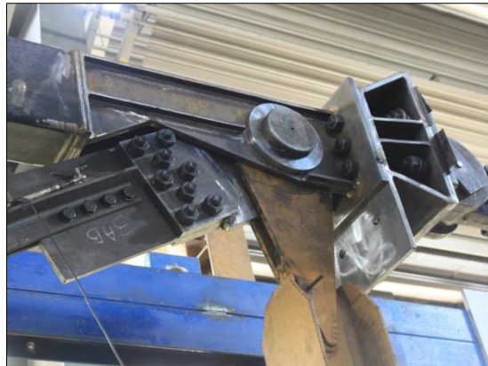
Figure 24. Beam-column joint in PF
