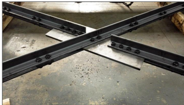
Figure 37. Steel mid-plate of the bracing system
