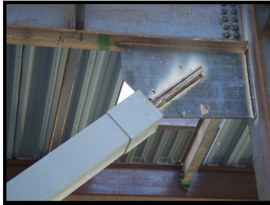
Figure 32. Angular gusset plate welded to the main members
