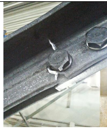
18. Crack propagation reaches horizontal flanges of the NE discontinuous diagonal (first tension peak of \pm 30 mm).
