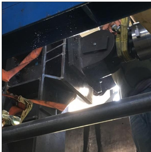
Figure 43. Fixing phase of the load cell to the MRF
