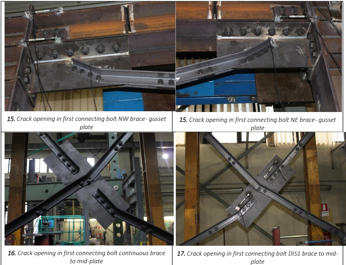
Figure 120. Crack opening at plastic hinges yet presented at frame nodes
