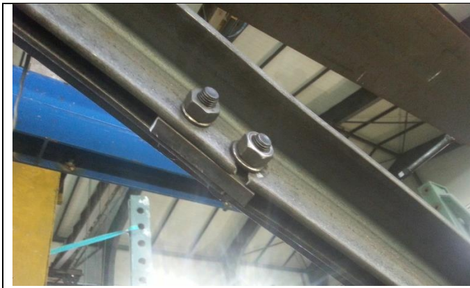
11. Crack opening at bolt of stitch plate of the NE discontinuous diagonal (first tension peak of \pm 20 mm).
