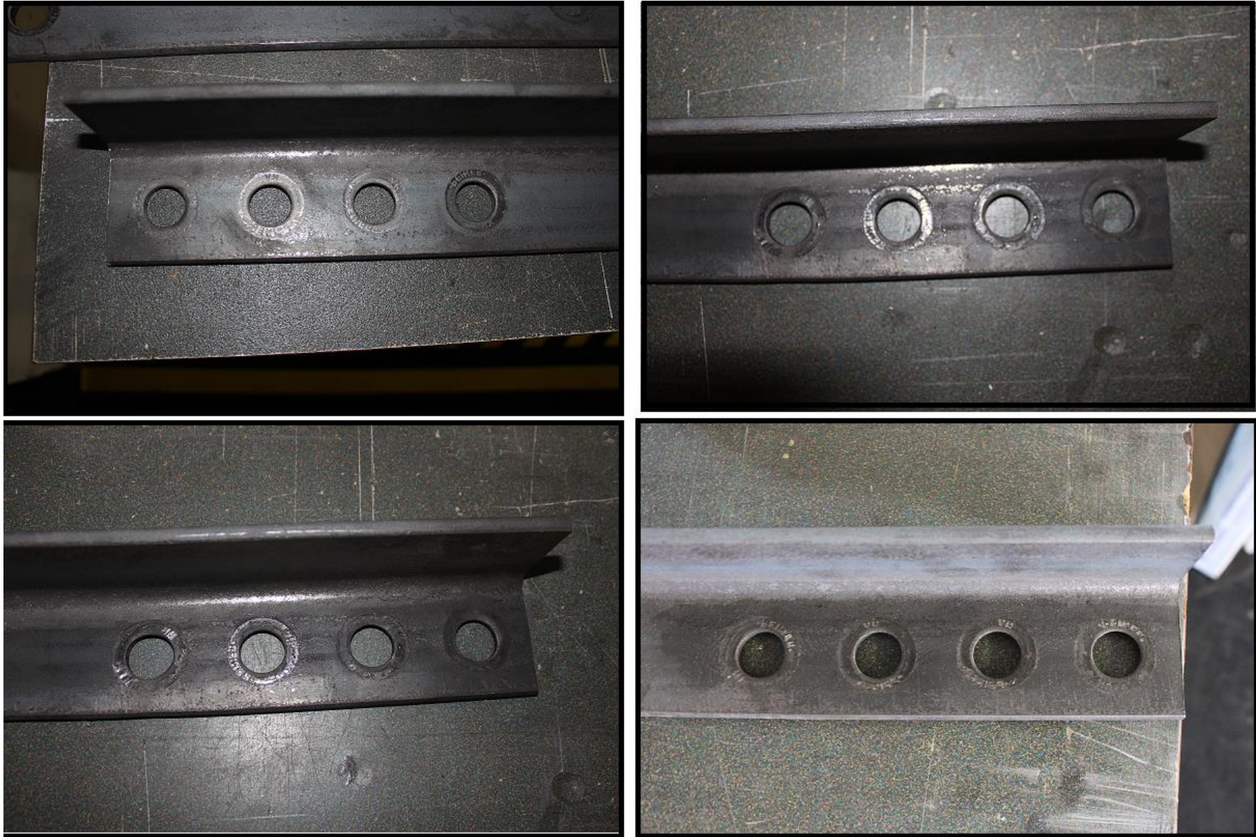
Figure 168. Bolt holes ovalization at brace joints ends
