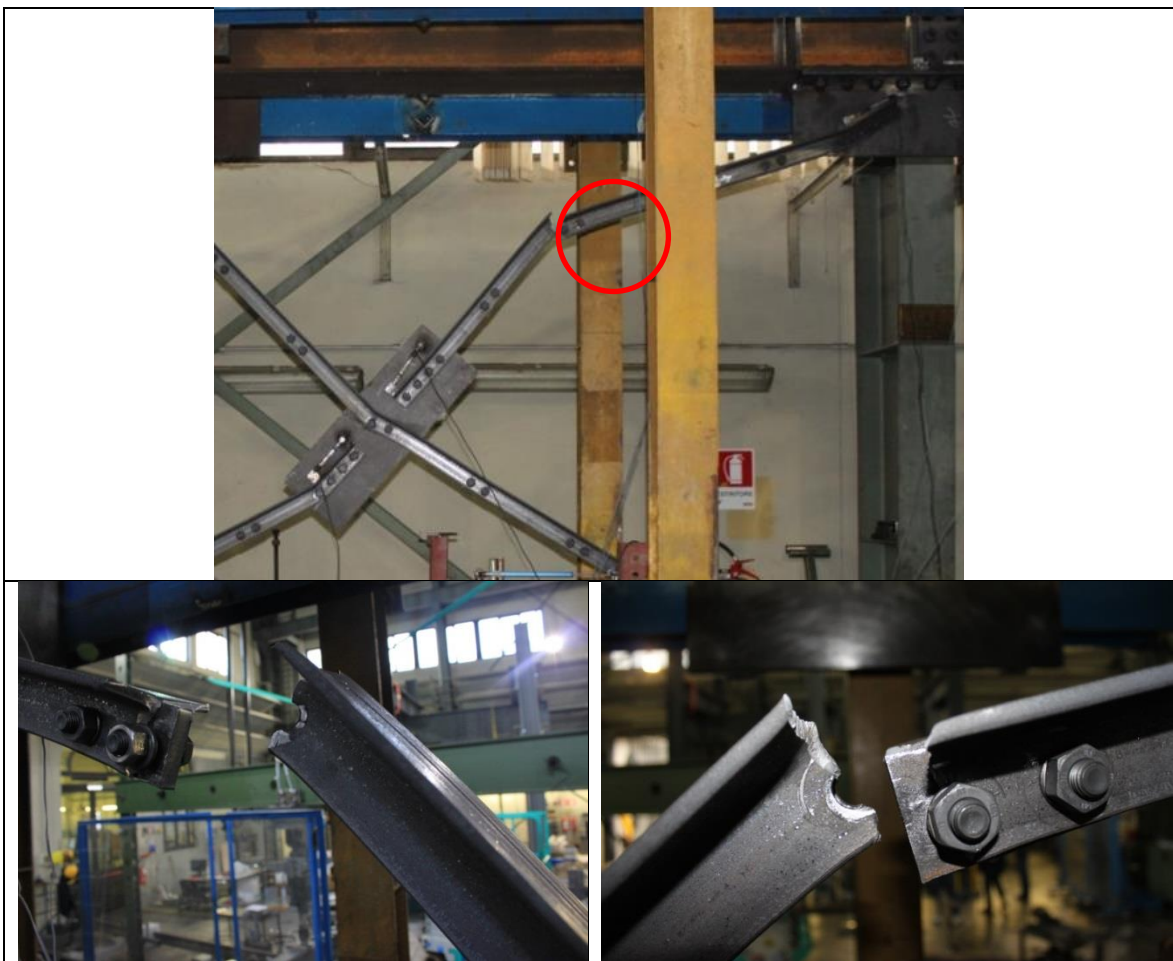
Figure 122. Failure along the stitch plate bolts in mid-span of the north-east discontinuous diagonal. (second frame tension peak of \pm 30 mm). Gross-section separation at mid-span of NE discontinuous brace. Cracks, initiated after plastic hinge formation, propagate.
