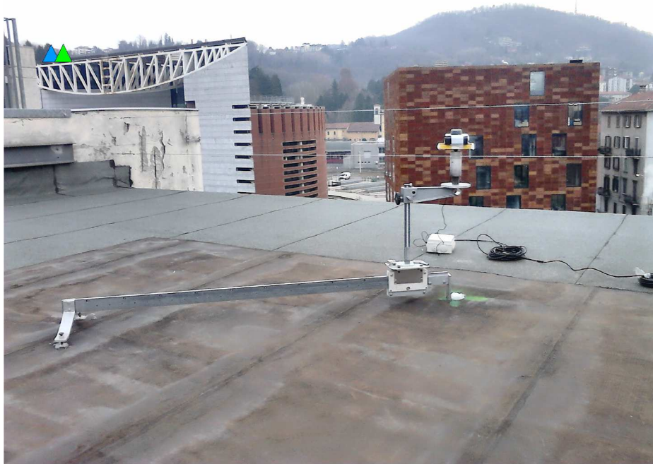
Figure 4.15 – The sliding device on Castelnuovo roof. In the upper left corner it is possible to see the position of reference stations (blue and green triangles)
