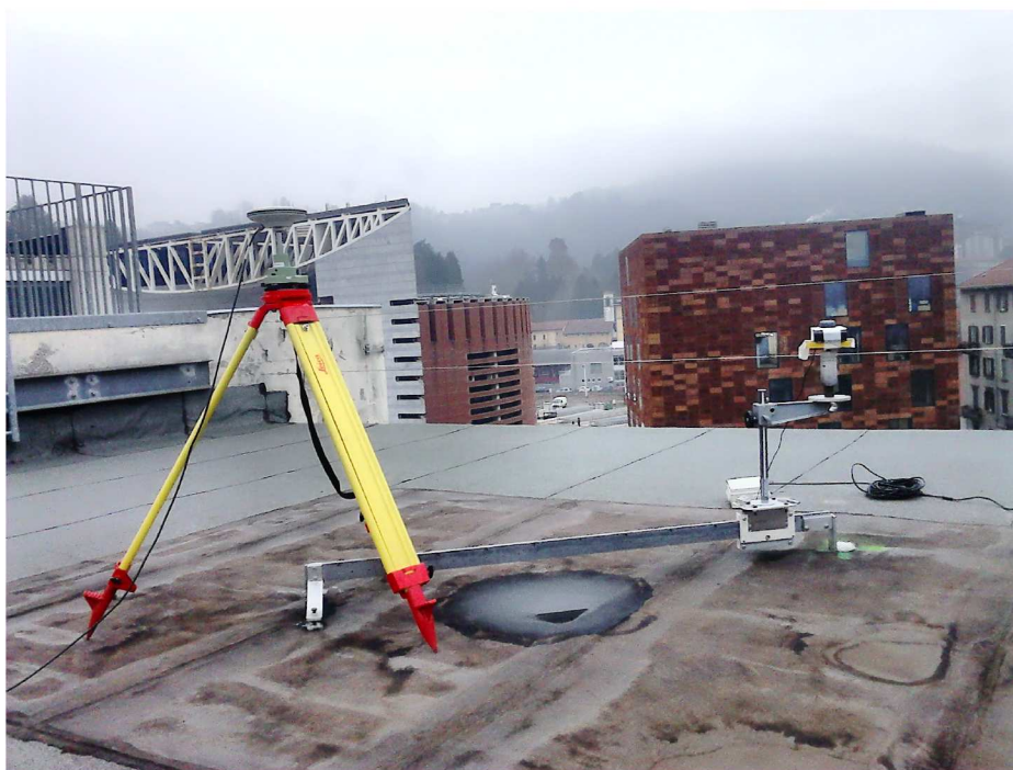
Figure 4.16 – Monitoring the roof stability with another geodetic receiver
