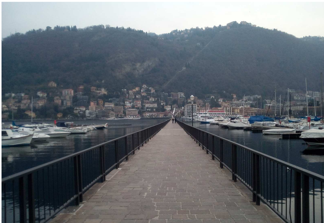
Figure 2.18 – Example of open area: breakwater Caldirola
