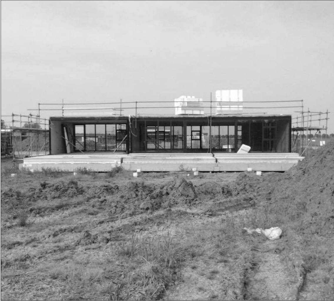
Figure 109: One building in Plot number 31. Photograph by author. Photograph by the author.
