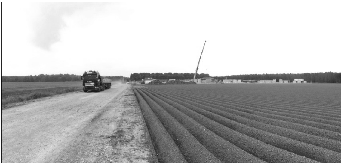
Figure 102: The first road built by private in Oosterwold. The road connects the preexisting street to plot number 31. This road is managed through an association of initiators. The association organizes actions and interactions, facilitates road maintenance and shares all the costs among initiators. Photograph by the author.
