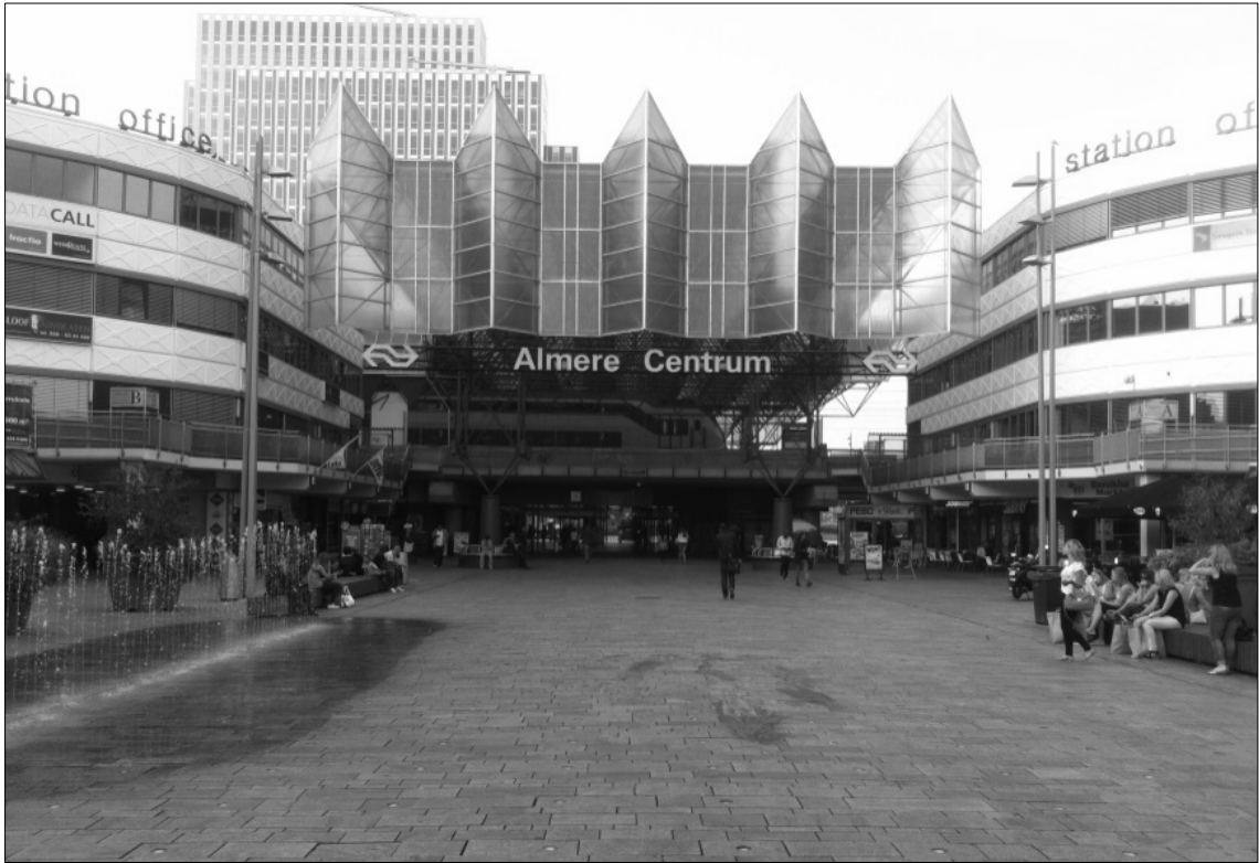
Figure 70: Almere Centrum, railway station. Photograph by the author.
