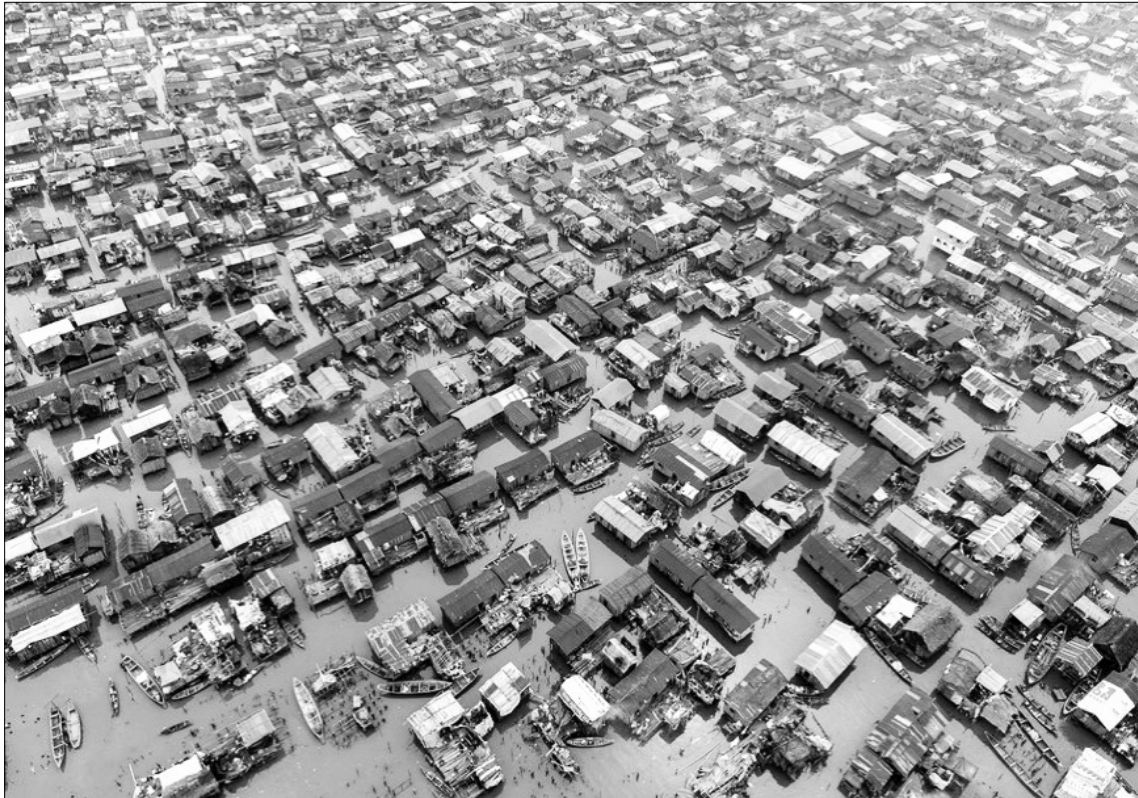
Figure 21: Lagos, Nigeria: an extreme case that shows the consequences of zero planning interventions (source: Gadanho, 2015).
