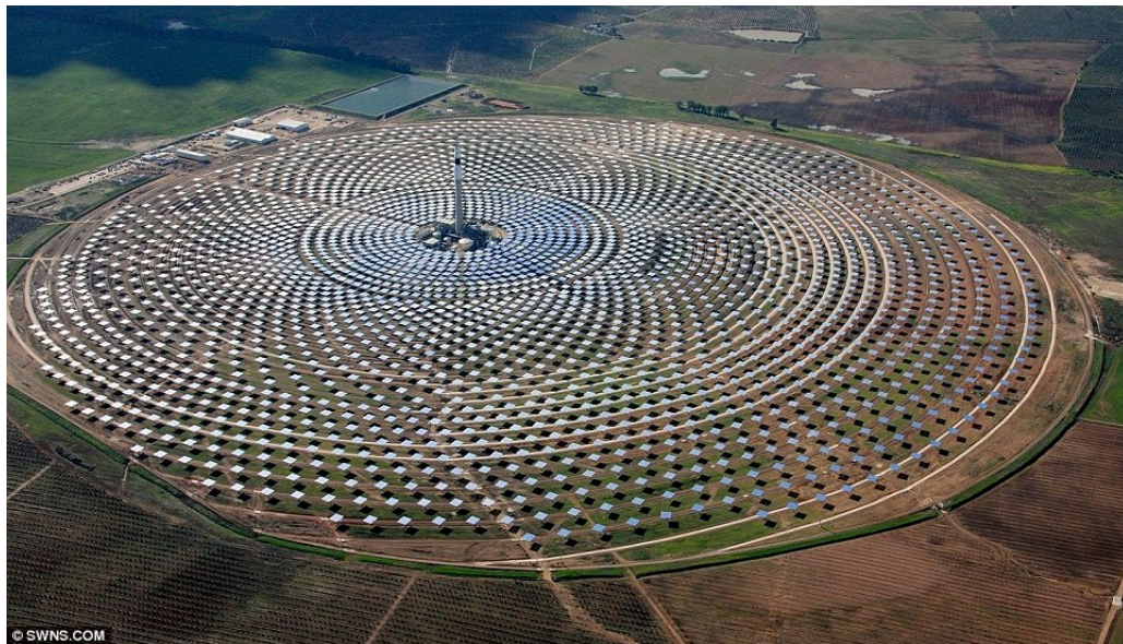
Figure 1.9: Gemasolar power plant.
