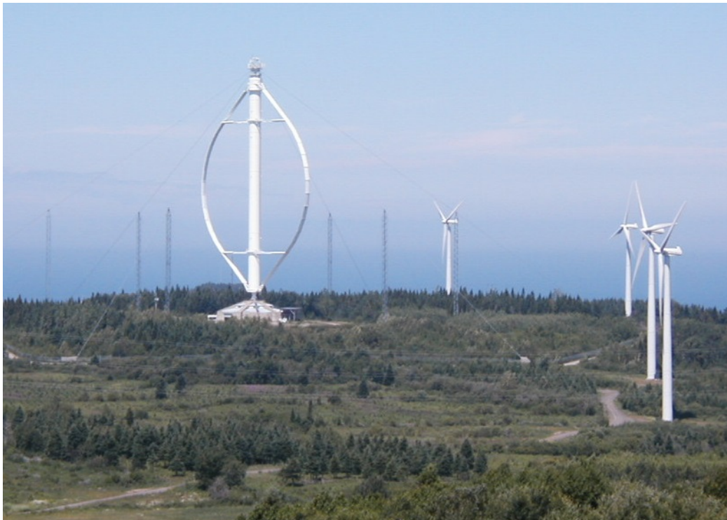
Figura 5.2: Turbina Éole a Cap-Chat , Quebec [16]
