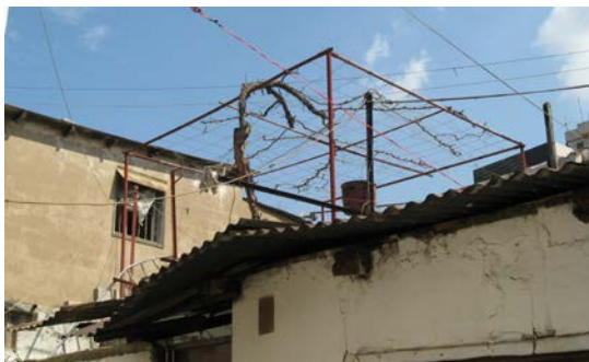
Figure 19. The roof as a communal space, a sitting area under a vineyard
