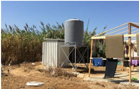
Figure 52. Water tank and toilet facilities
