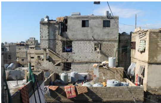
Figure 27. Vertical expansion of houses in Shatila
