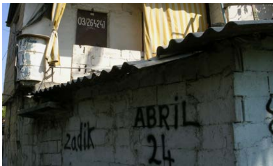
Figure 14. Addition of floors and zinc roofs
