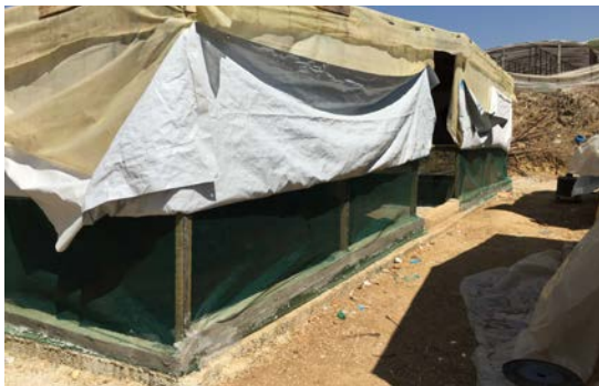
Figure 42. Shelter for Syrian refugees in Bebnine: poured concrete on the floor, wooden posts and tarpaulin
