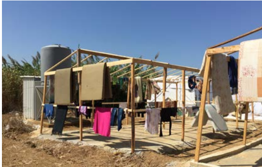
Figure 44. First phases on construction of tents in Bebnine
