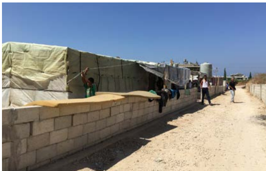
Figure 45. Parapet delimitating the space of the camp
