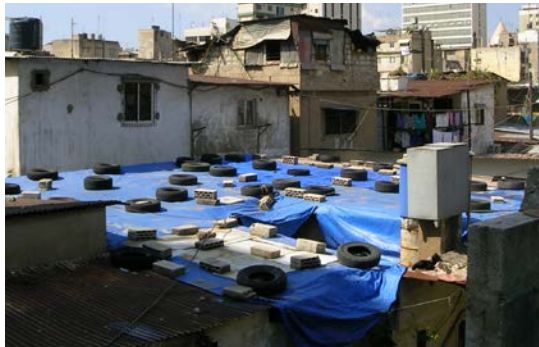
Figure 18. Wheels placed on the zinc roof to stabilize them in the rainy days
