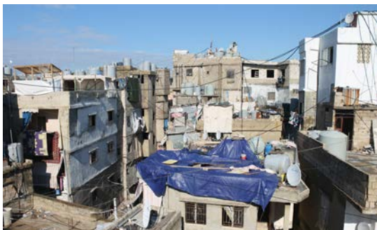
Figure 32. Tarpaulin added for waterproofing purposes on the roof
