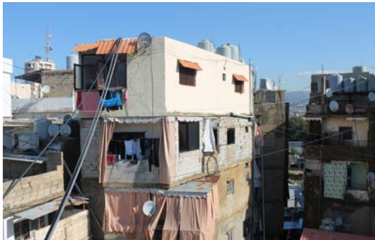
Figure 30. Unplanned addition of spaces and floors on top of original family house
