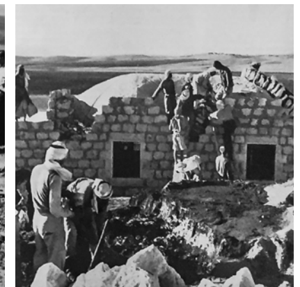
Figure 26. The plans settled, the refugee masons work on the buildings of the Beit Qad agricultural cooperative.
