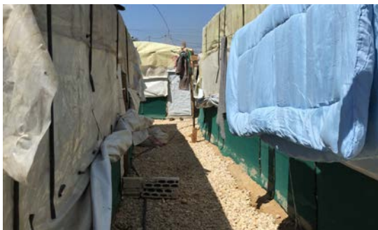
Figure 43. Alleys between tents covered with gravel to prevent flooding
