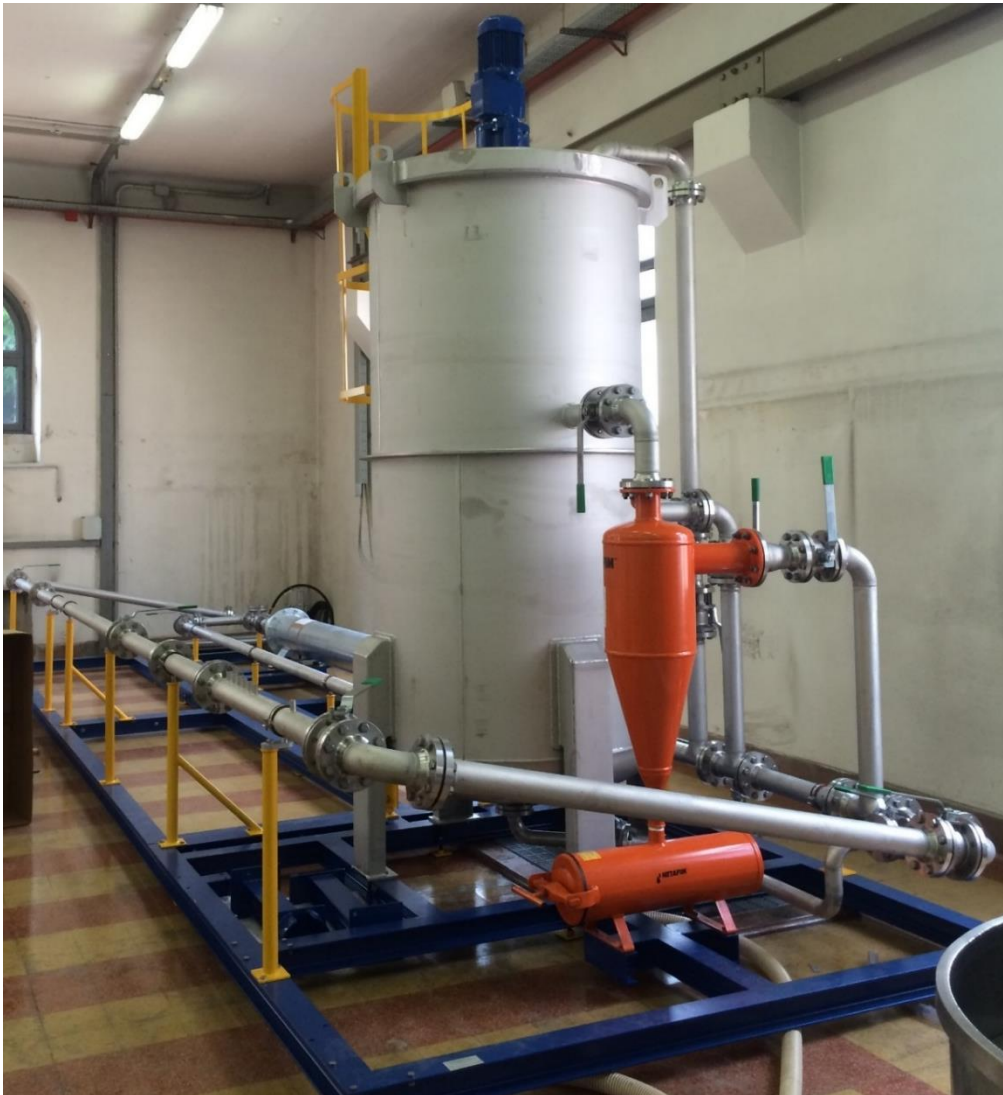
Fig. 79 Erosion Loop system at G.Fantoli Laboratory
