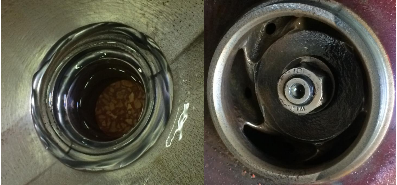
Fig. 21 Entrance of the water and impeller
