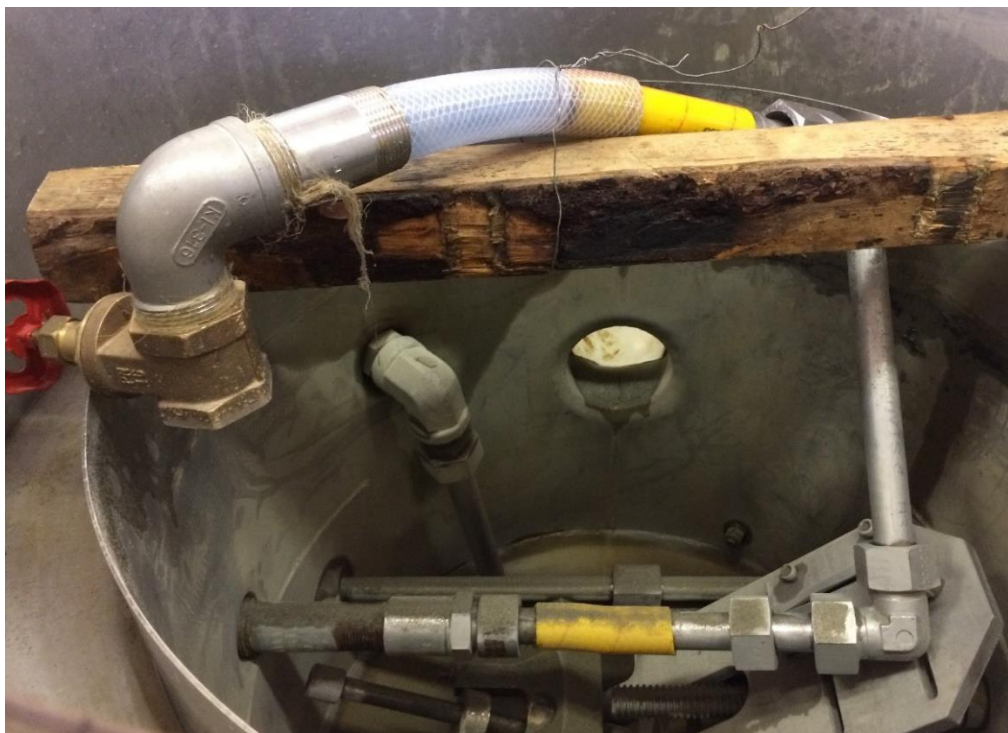
Fig. 33 Second configuration in the filling set up: all the pipes are fixed
