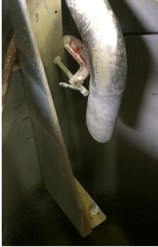
Fig. 28 Exit of the flux from the upper tank: place for concentration sampling
