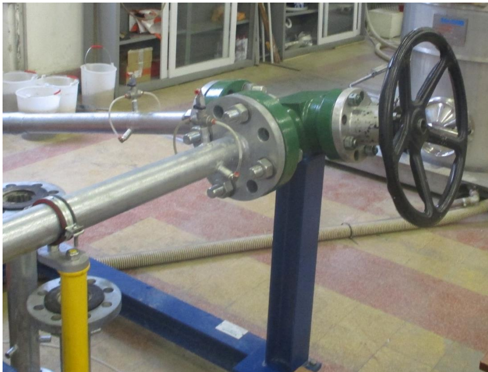
Fig. 80 Choke Valve installed on the loop system.
