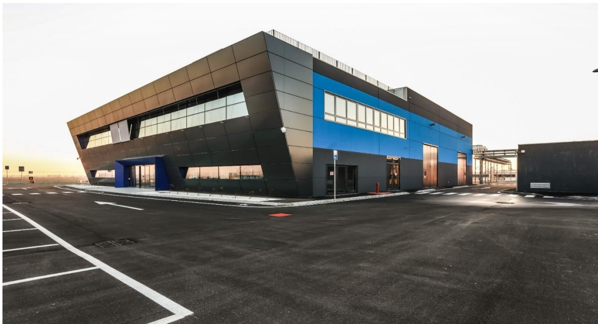
Figure 14 Avio Aero AM plant
