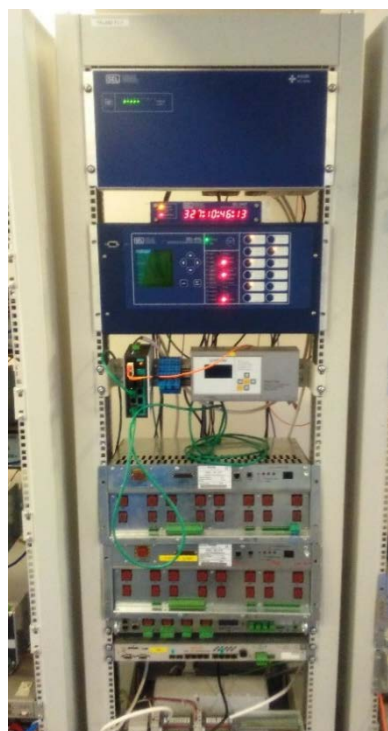
Figure 48 From the top: the AXION PMU model, the SEL 2407 clock, the SEL 411L PMU model.
