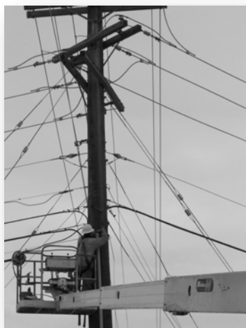
Figure 13 Dual feed and underground transition on distribution feeder.
