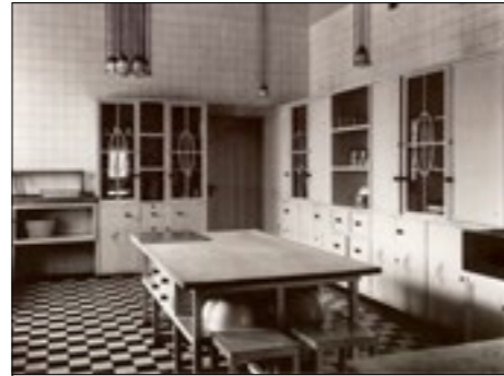
1905-11 Joseph Hoffmans kitchen in the Palais Stoclet, Traditional large working table, all white and covered with tiles up to ceiling for hygienic reasons.
