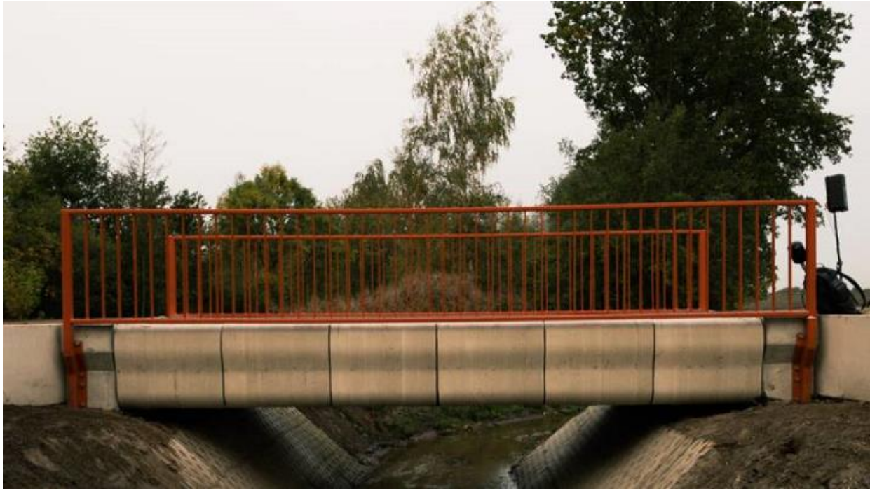
Figure 45. 3D Printed Pedestrian Bridge – Gemert, Netherlands ( 3dprint.com ).
