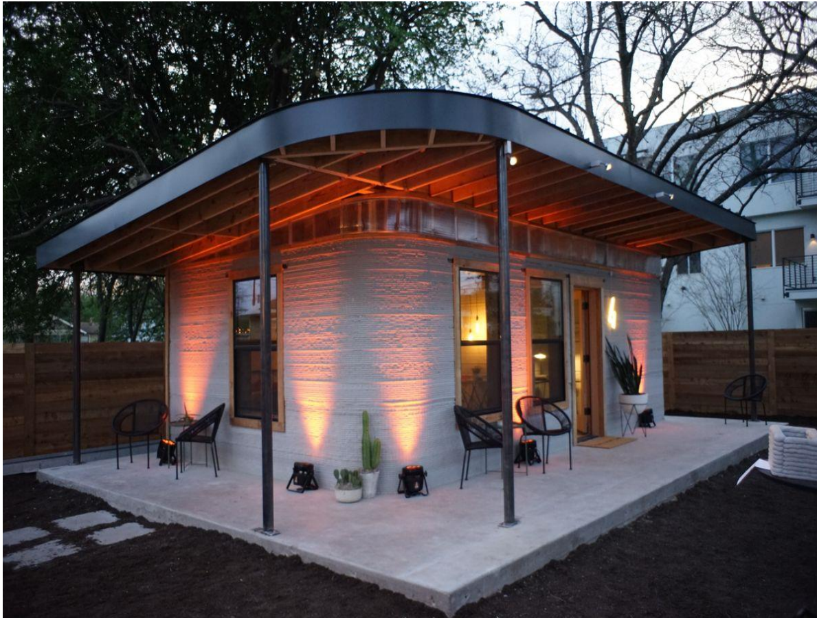
Figure 19. Cheap Housing Using Concrete 3D Printing ( theverge.com ).
