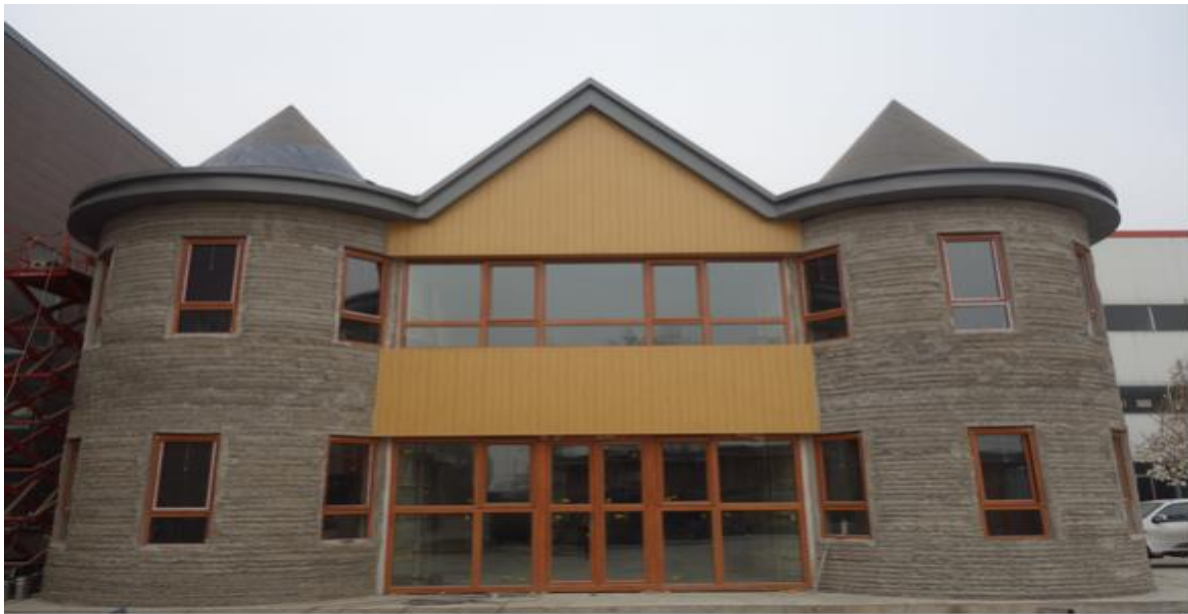
Figure 35. Two-story 3D printed house ( 3dprint.com ).
