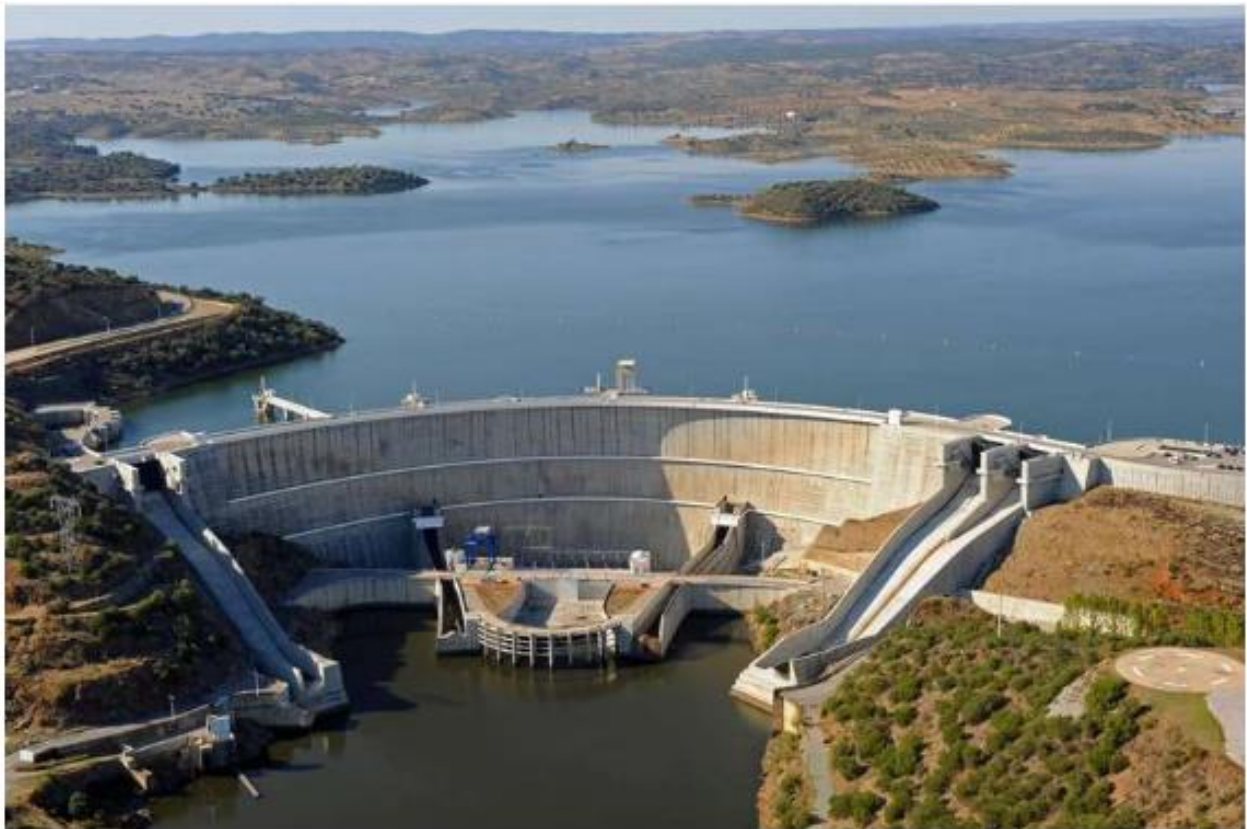
Figure 26 Alqueva Pumped Hydroelectric Storage Plant, Portugal
