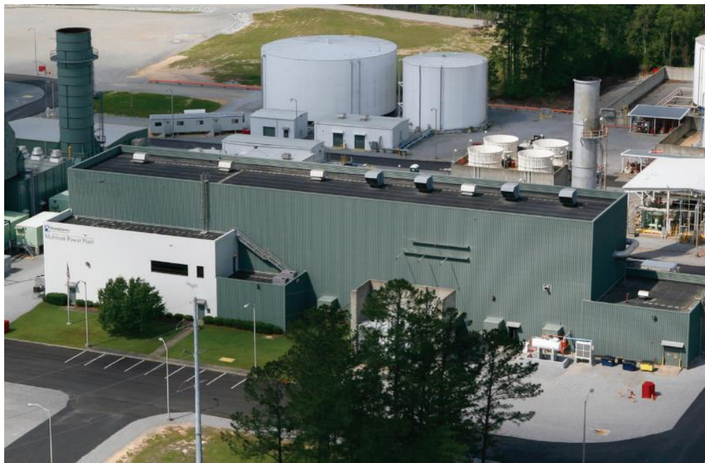
Figure 22 McIntosh CAES Plant, Alabama U.S.A., Nominal power 110 MW, Discharge duration 26 hours
