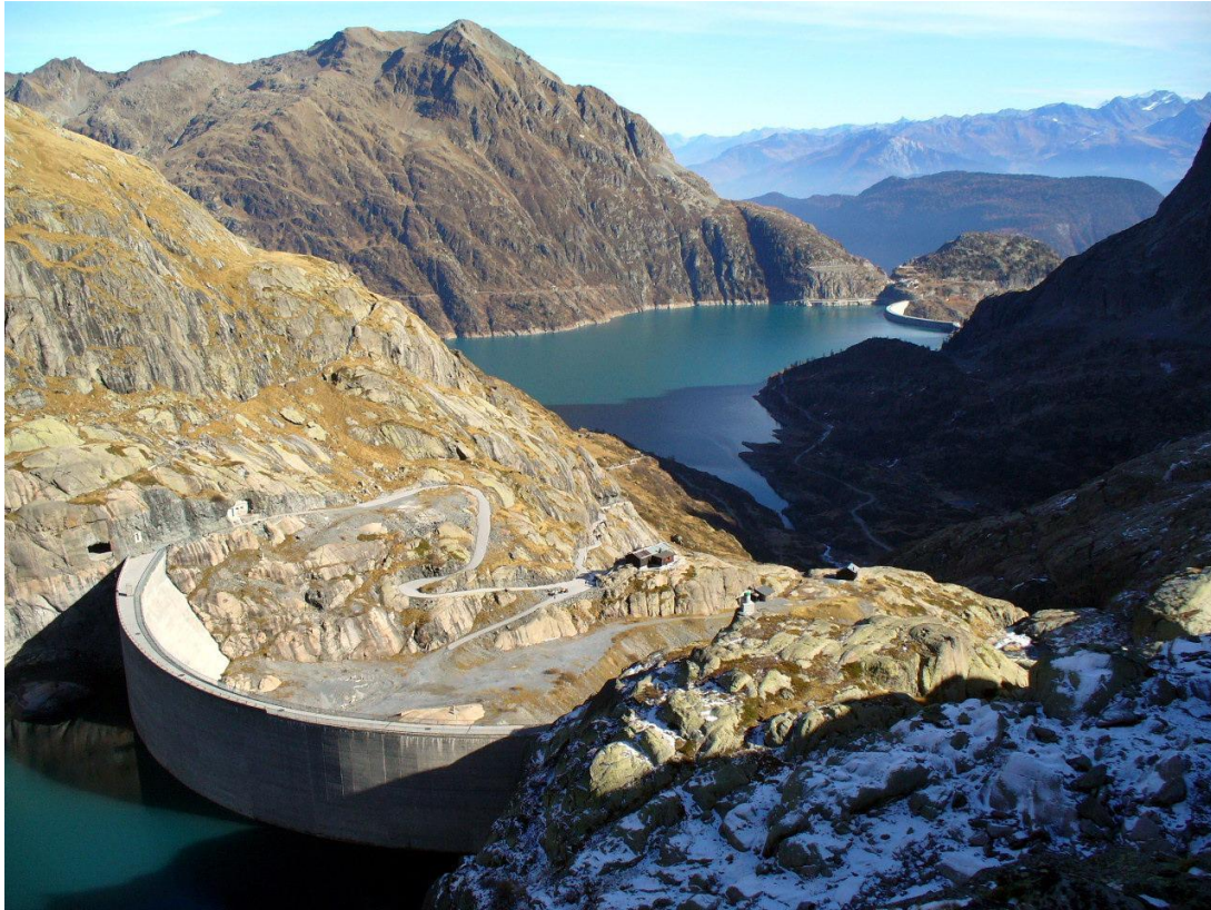
Figure 27 Nant de Drance PHS, Switzerland 900 MW nominal power
