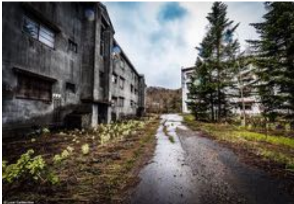
Figure 3.7: Yubari Abandoned Building (Source: https://www.dailymail.co.uk/news )
