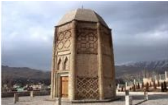
Figure 4.32: Shebly tower (Source: https://tripyar.com )
