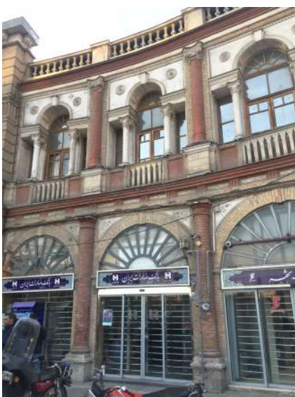
Figure 88: Hassan Abad Square building facade (Self Elaboration)
