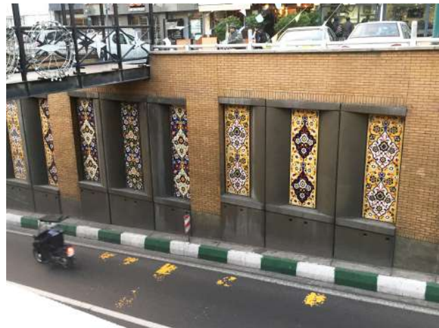
Figure 90: Facade of the underpass (Self Elaboration)
