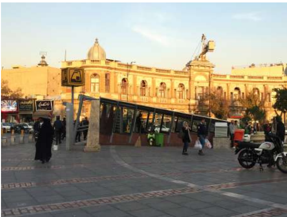
Figure 85: Hassan Abad Square metro station (Self Elaboration)
