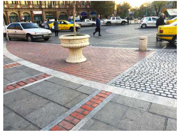
Figure 84: Hassan Abad Square pavement (Self Elaboration)
