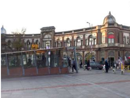
Figure 91: Hassan Abad Square pavement (Self Elaboration)
