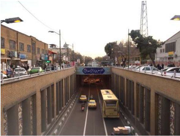
Figure 83: Hassan Abad Square underpass (Self Elaboration)
