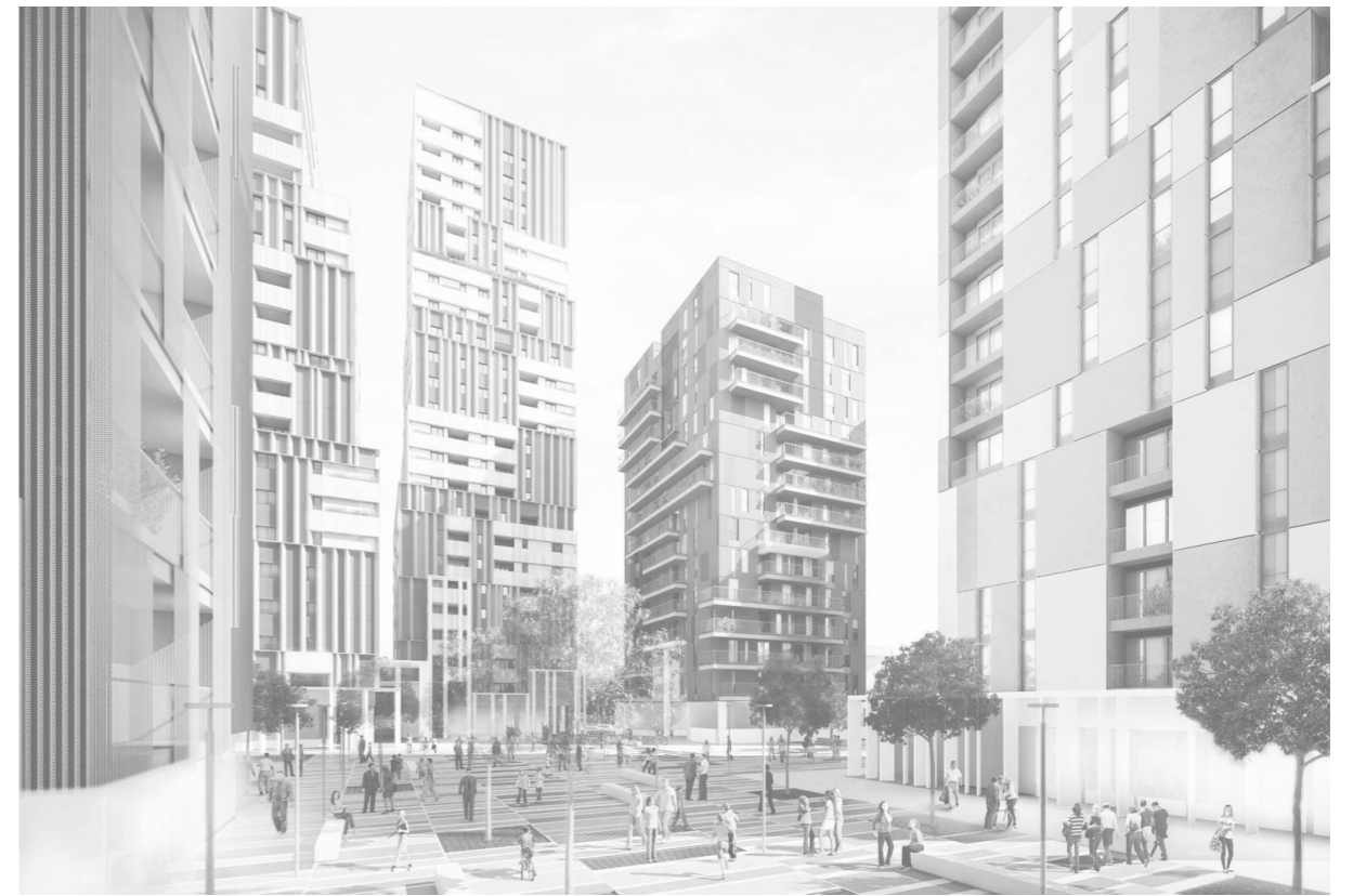
Figure 60. Cascina Merlata Housing District exterior view (CZA, 2011)
