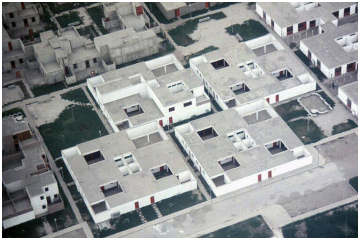
Figure 39. PREVI Low Cost Housing aerial view (James Sterling, 1969)
