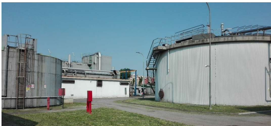
Figure 3.2 The WWTP under study: on the left, the pre-thickening unit; on the right, one of the anaerobic reactors
