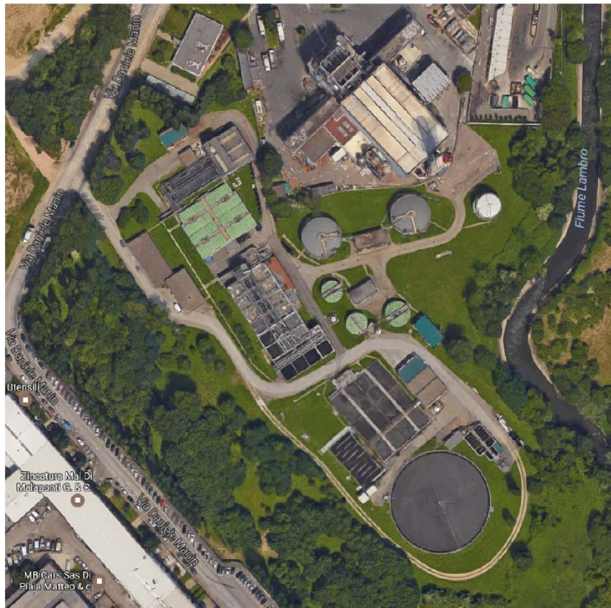
Figure 3.1 Satellite view of the WWTP under study
