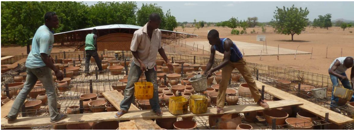
Figure 14. Gando School Library. Construction process. Source: (Kéré Architecture, 2020)
