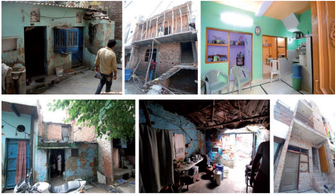
Figure 24. Before and after of two houses during the pilot. Source: (van Noppen, et al., 2011)
