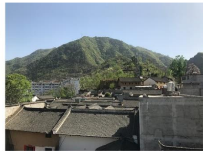
view on the top of building
