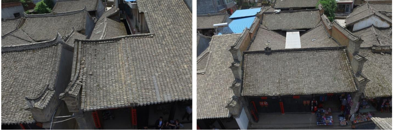
Fig. 1.28 Fire wall of Fenghuang Ancient Town (Source: drone survey made during the PoliMi-XAUAT Workshop, May 2018)
