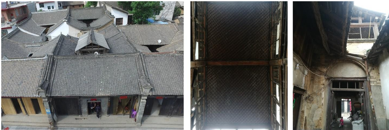
Fig. 1.29 Lantern-like transparent roof of Fenghuang Ancient Town (Source: drone survey made during the PoliMi-XAUAT Workshop and author, May 2018)
