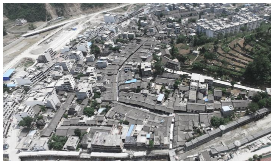
Fig. 1.18 2018 Fenghuang Ancient Town (Source: Drone survey made during the PoliMi-XAUAT Workshop, May 2018)
