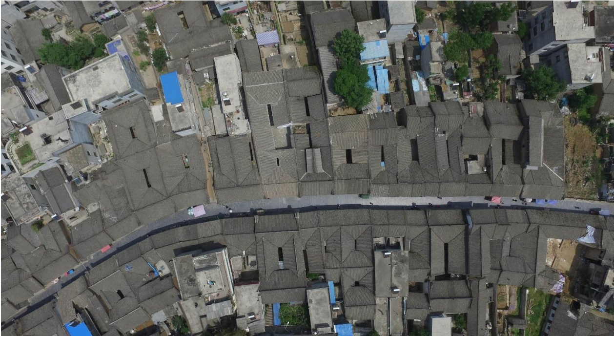
Fig. 1.24 The 'front store, back house' and 'narrow courtyard' type (Source: drone survey made during the PoliMi-XAUAT Workshop, May 2018)
