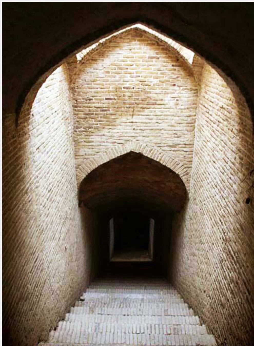
Figure 134: Giv Water Reservoir, stairway and access to Pashir, photo by Faride Hassani
