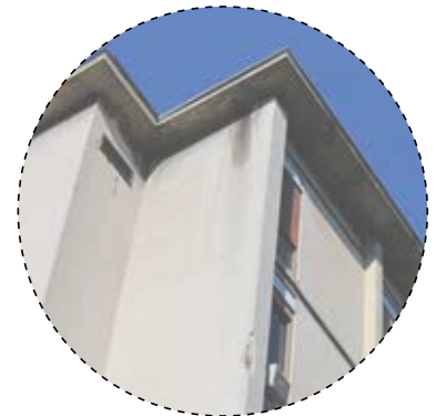
Fig. 02.68 Picture of Convitto's roof
