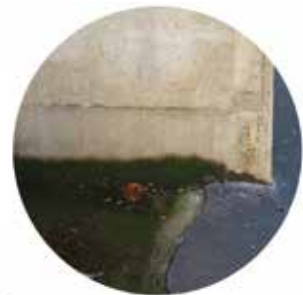
3 Fig. 02.96 Biofilm growing on the ground and through the facade
