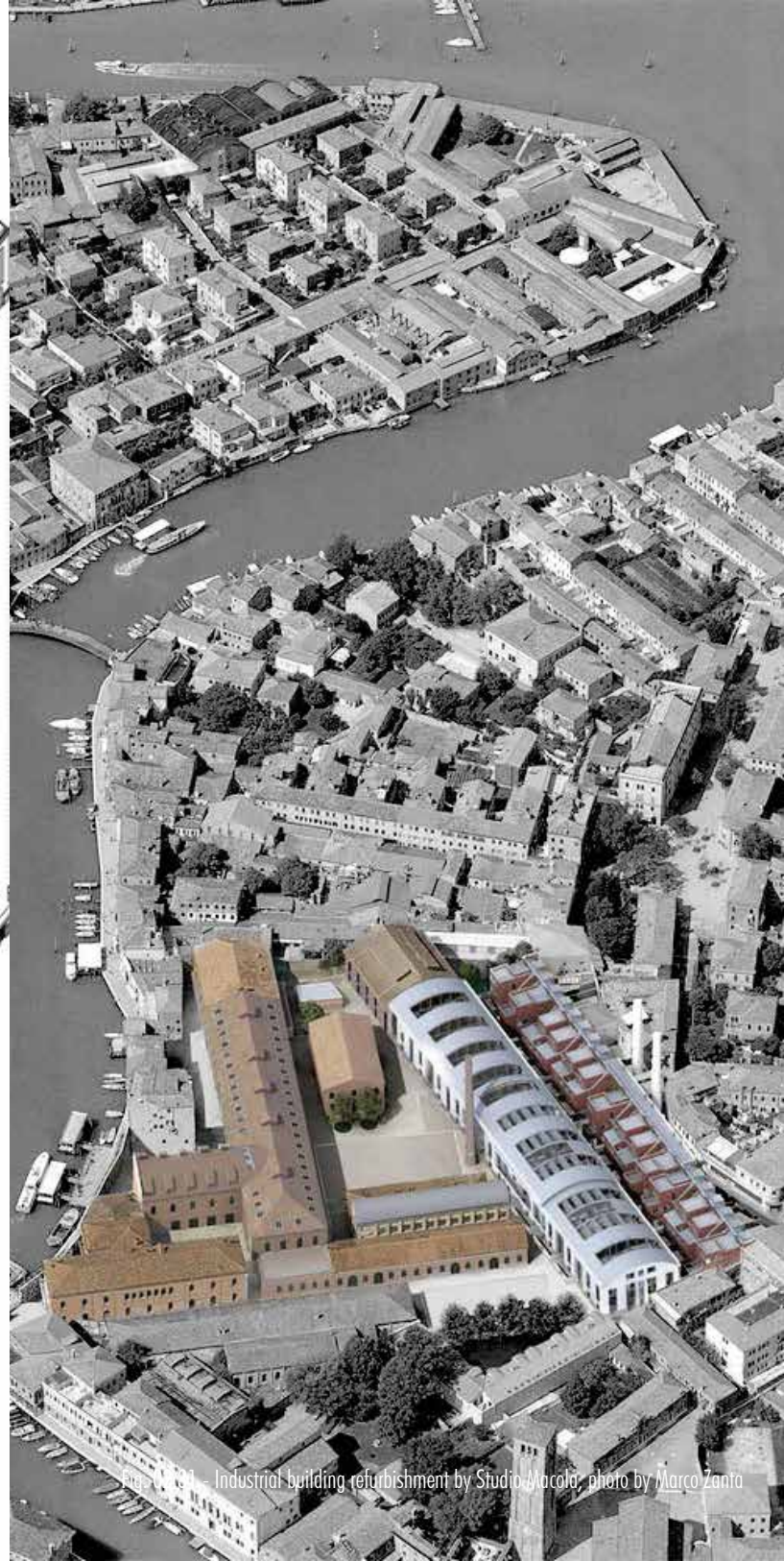
Fig. 2.30 - Industrial building refurbishment by Studio Macola
