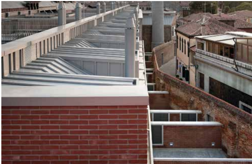
Fig. 02.32 - Industrial building refurbishment by Studio Macola
