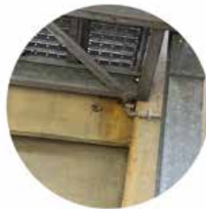
2 Fig. 02.95 Rust staining of metal parts, due to iron oxides driven by water
