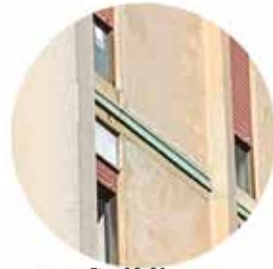
2 Fig. 02.91 Patinated copper elements and painting films peeling off from the plastered facade
