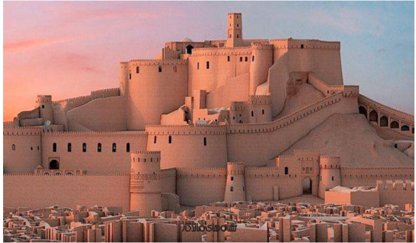
Figure 4-1- Masonry walls with high thermal inertia. Arge-e-Bam, Kerman/Iran
