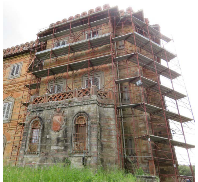
FIGURE 34. SIDE VIEW OF SAMMEZZANO, PICTURE BY ANGELA FONTANA, 2021
