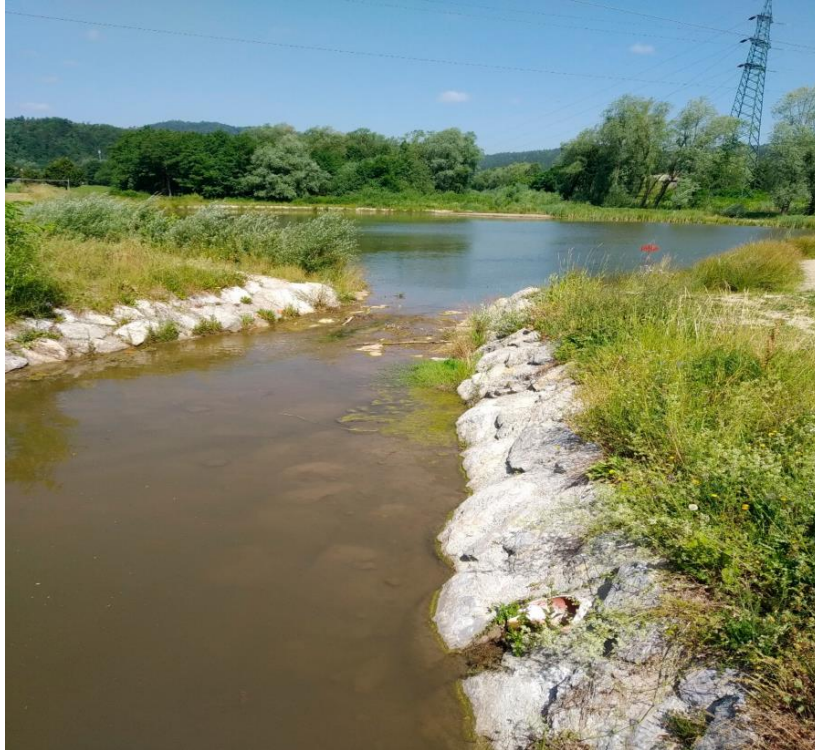
Figure 8: Upstream reservoir in Glinščica River basin 11
