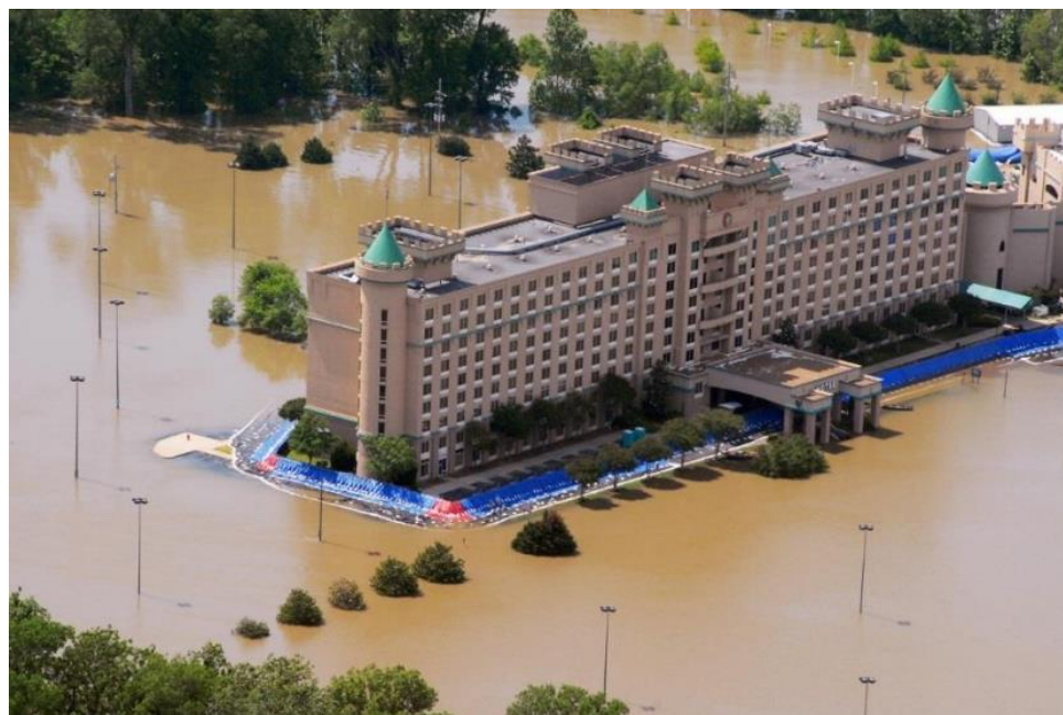
Figure 13: Use of temporary cofferdam implemented by PORTADAM Company 16
