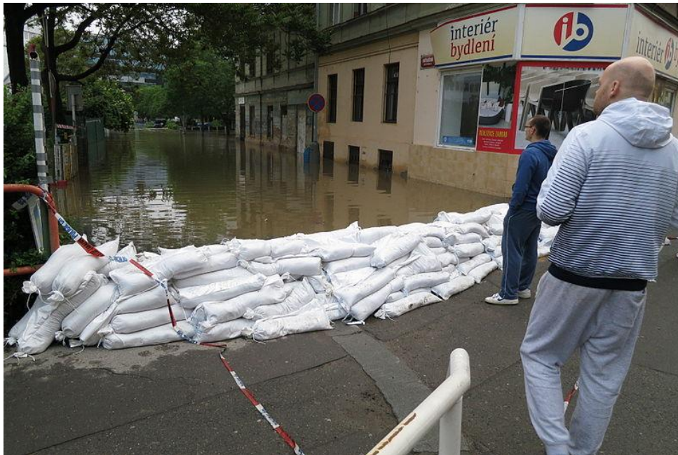
Figure 12: Use of sandbags during the flooding in Prague, 2013 15
