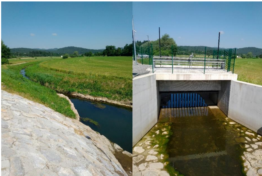
Figure 9: Outflow structure and downstream of the Glinščica River basin 12
