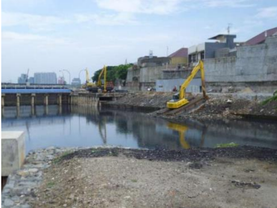
Figure 10: Water retention reservoir refurbishment and expansion in northern part of Jakarta. 13
