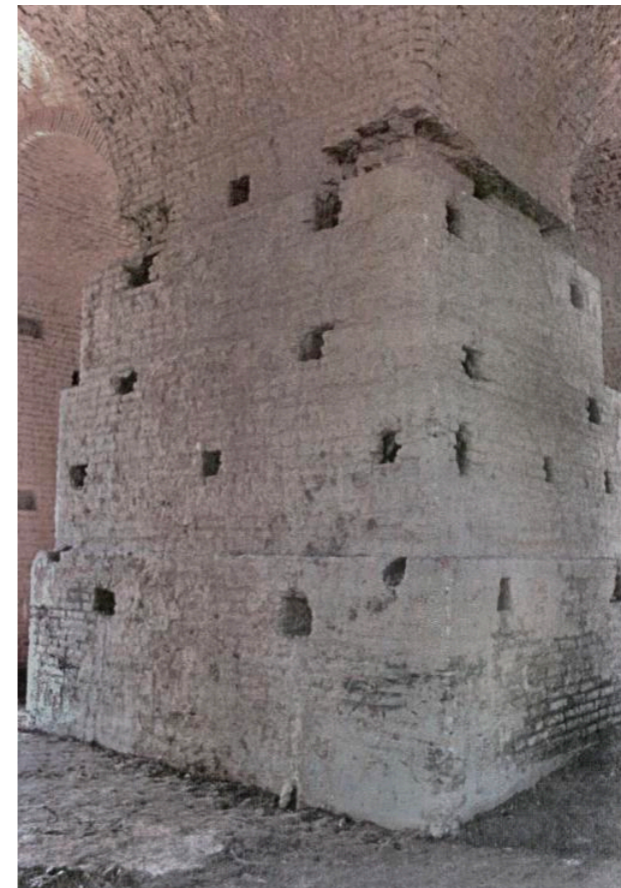
The pillars of the pavilion inside the lake The holes inside can control the water stream
