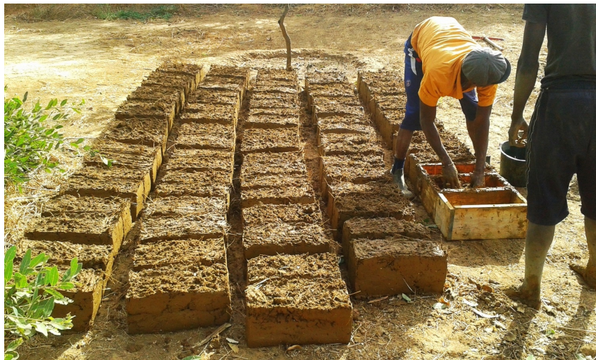
Figure 2.1: Straw reinforced mud-brick production
