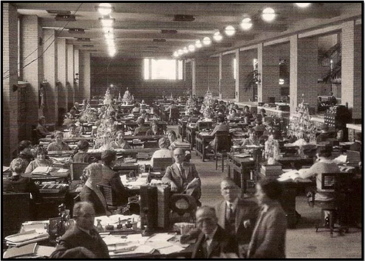
Figure 1 The Larkin Administrative Building in the 1900s
