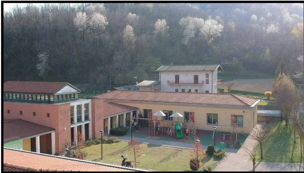
Figure 29 Aerial view1 from the North-east
