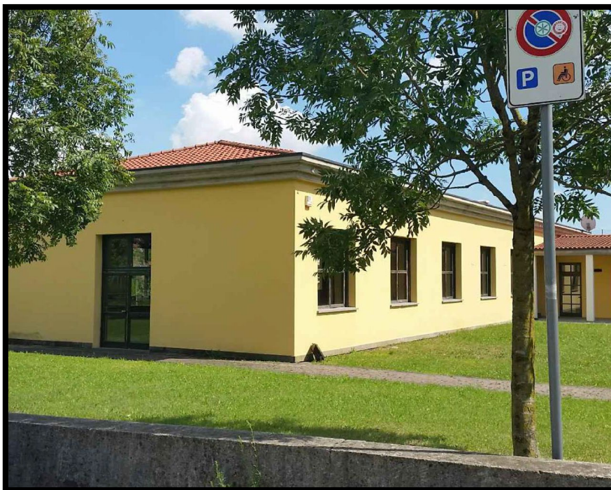
Figure 39 View 4- Current state of the Building
