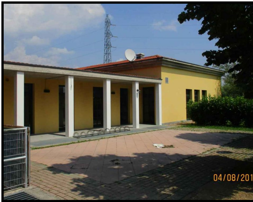
Figure 38 View 3- Current state of the Building
