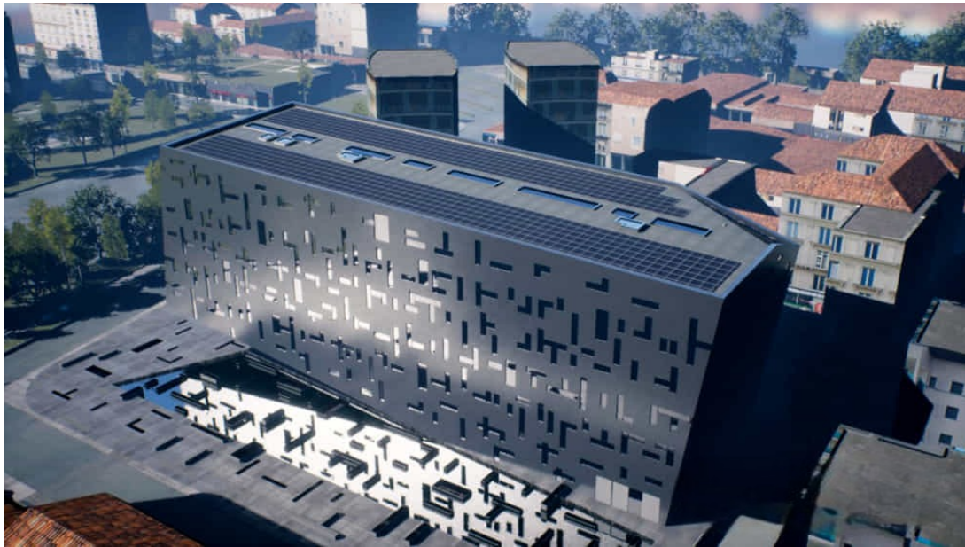
Figure 6.1: Roof View of the building
