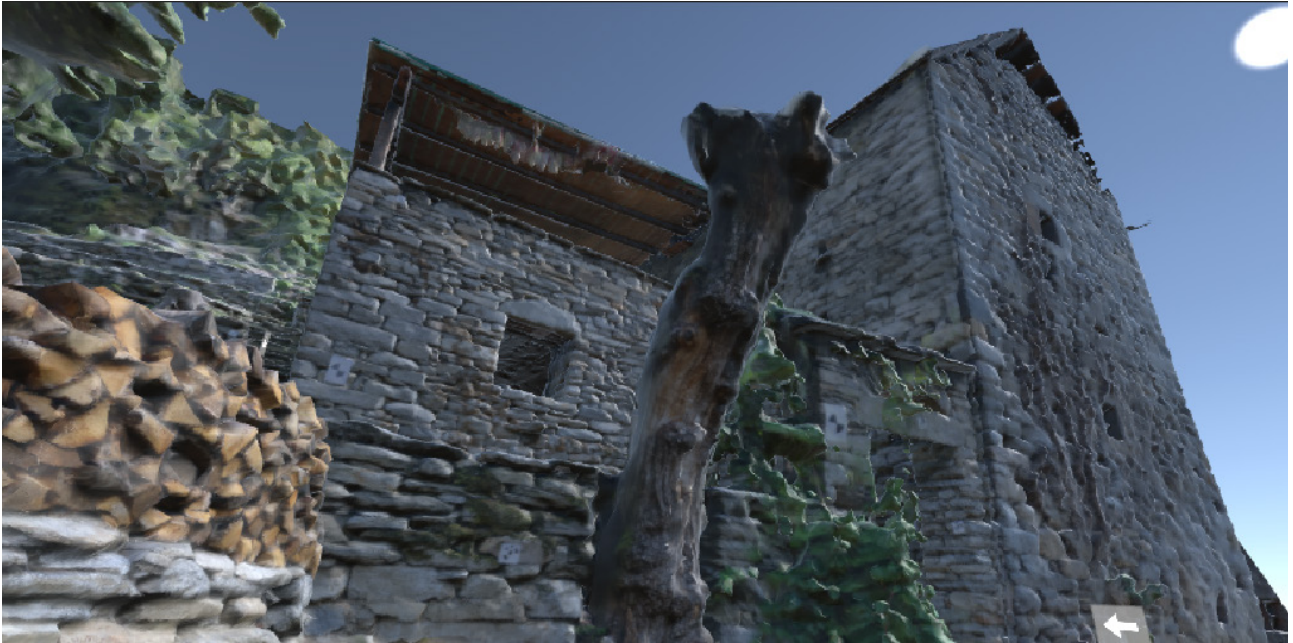
Figure 3.34 Casa dell'Affresco, looking from the Balma House. (Elaboration by the authors)
