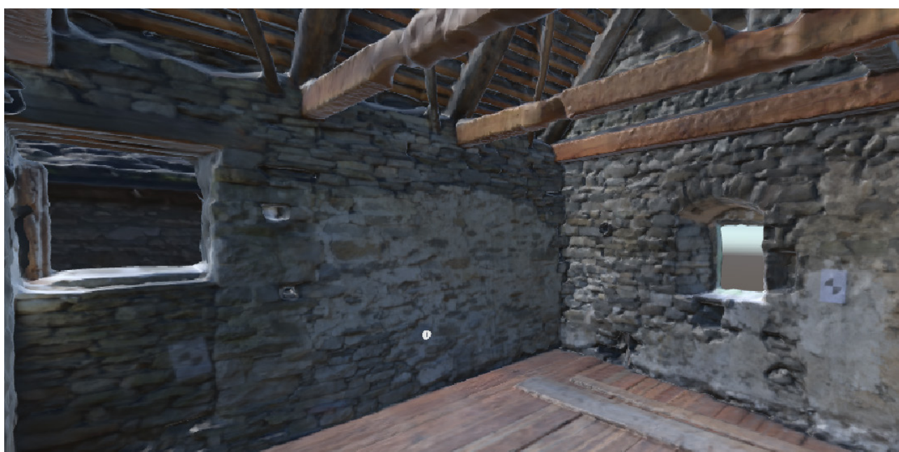
Figure 3.37 Room inside of the Casa dell'Associazione in 2017. (Elaboration by the authors)
