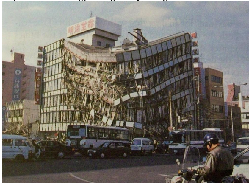
Figure 1. The collapse of a steel building during Kobe, Japan earthquake in 1995 [3]
