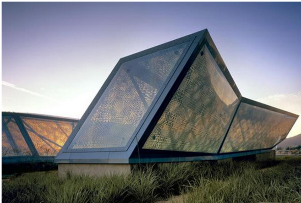
Illustration 138 Configuration of three foils with sun shading system foil (extracted from VECTORFOILTEC 111 )
