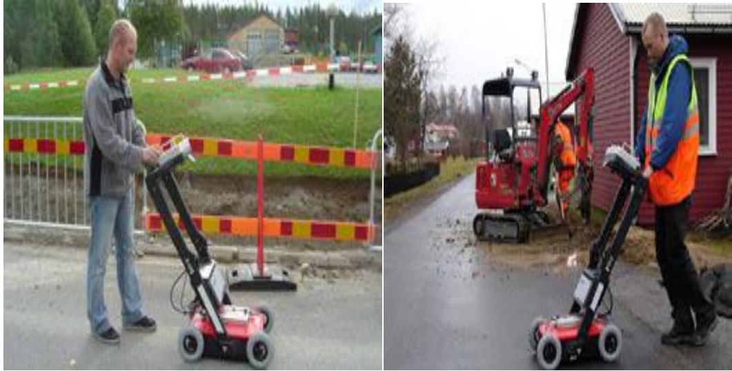
Figure 2.37: MALA Easy Locator investigating the subsurface.
