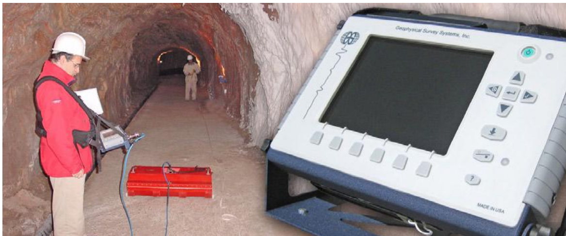
Figure 2.25: SIR-300 being used to inspect a tunnel.
