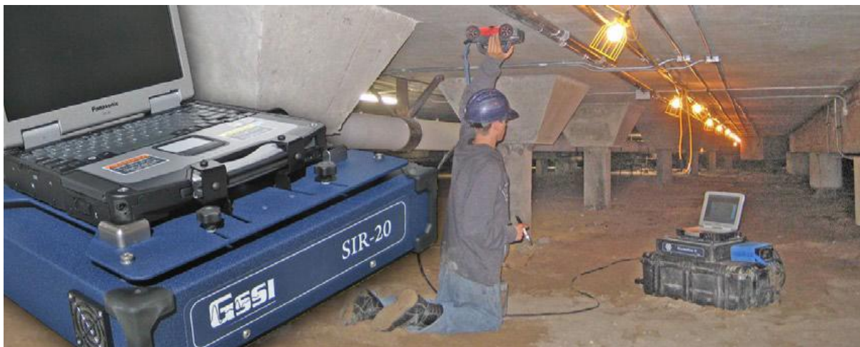
Figure 2.23: GSSI SIR-20 inspecting a bridge deck.
