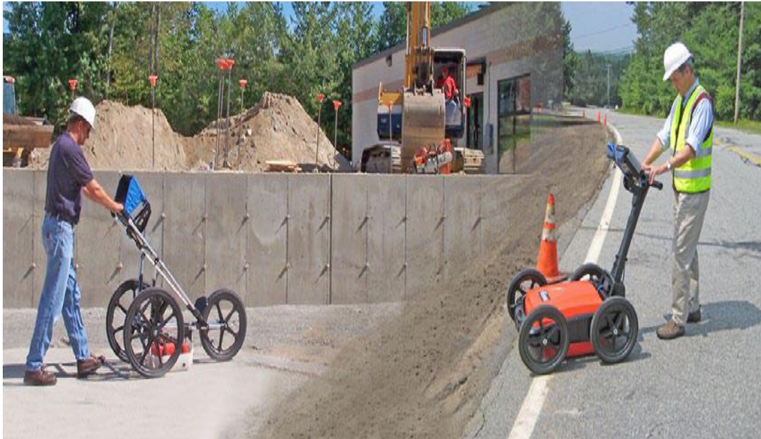
Figure 2.33: UtilityScan locating and mapping underground utilities.
