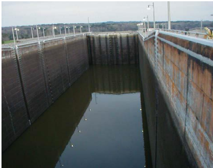
Figure 2.13: A lock at the Walter F. George Dam.
