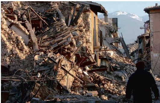
Figure 1-3: Aftermath of L'Aquila earthquake (April 2009)
