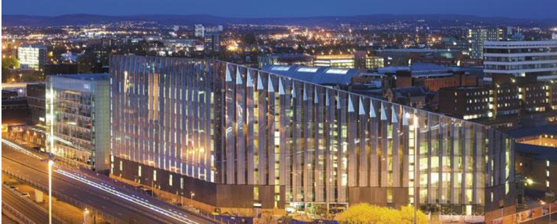
Figure 3-3: Global view of the Manchester Metropolitan University building (Courtesy of Permasteelisa S.p.a.).
