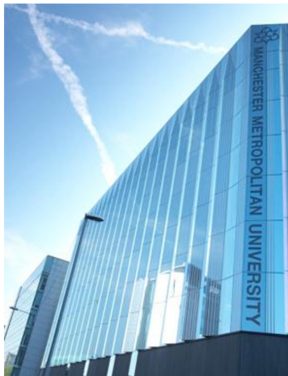
Figure 3-2: Outside view of the Manchester Metropolitan University façade (Courtesy of Permasteelisa S.p.a.).
