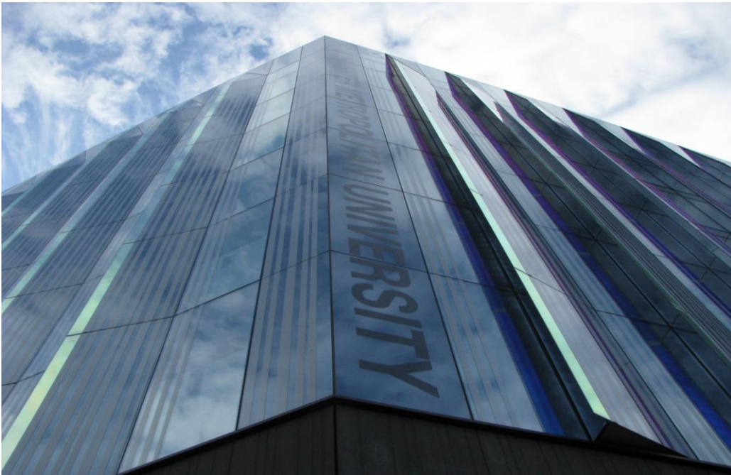
Figure 3-1: Outside view of the Manchester Metropolitan University façade (Courtesy of Permasteelisa S.p.a.).
