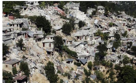
Figure 1-4: Aftermath of Haiti earthquake (January 2010)
