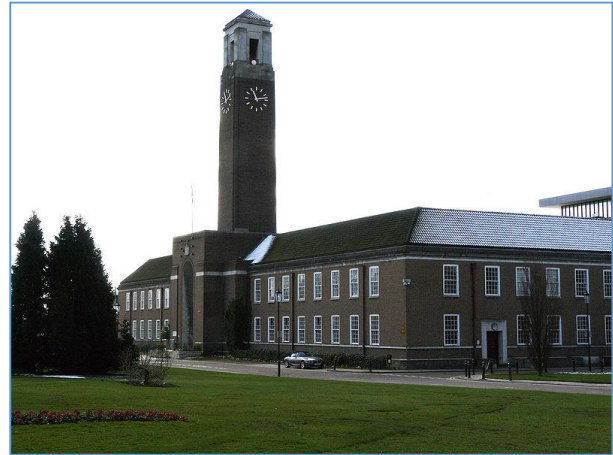
Figure 16 Salford Civic Centre, in Swinton
