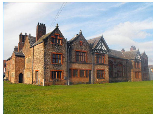
Figure 51 A view of the west side of the west wing, with the Great Hall in the middle
