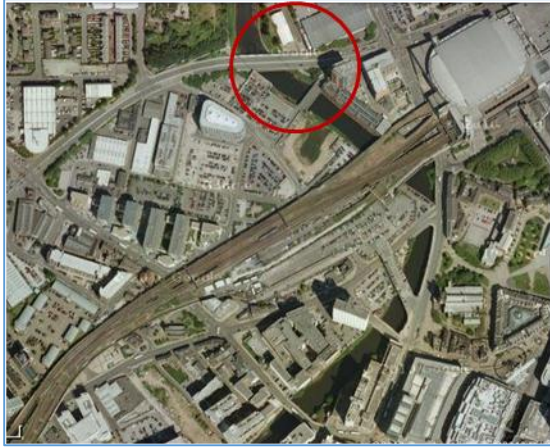
Figure 79 The Trinity Way Bridge and The New Bridge St. locality
