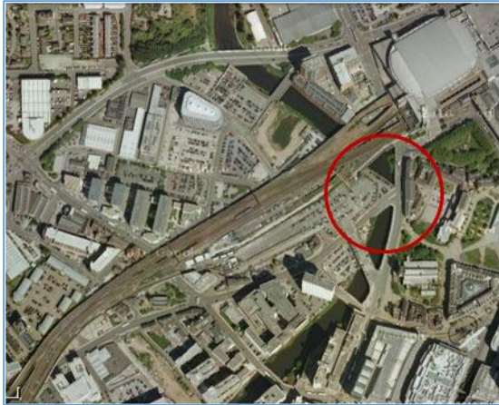
Figure 81 The Chapel Street Bridge locality.
