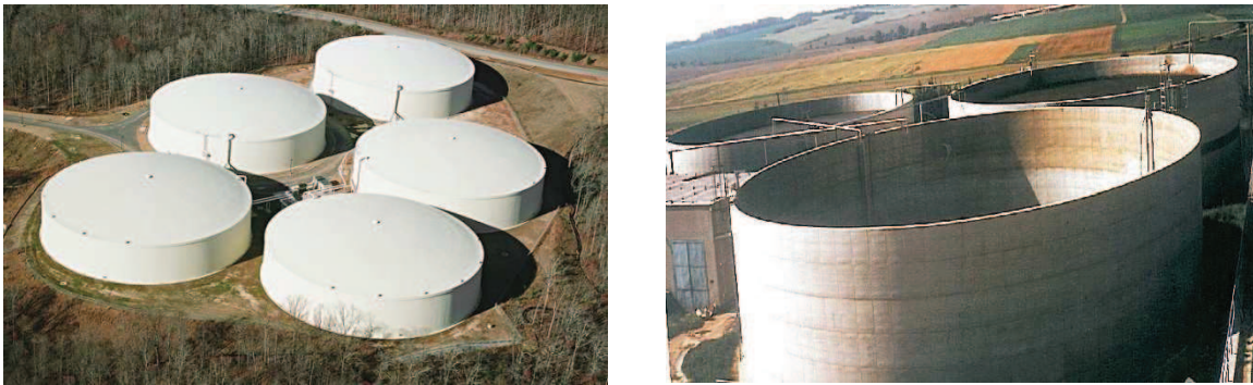
Figure 2: Concrete storage tanks.
