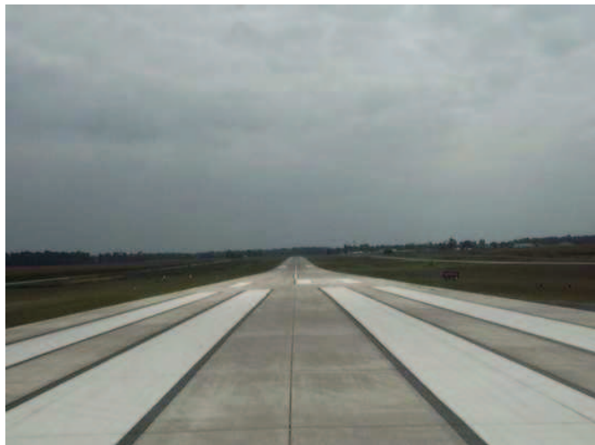
Figure 4: Concrete airport runways.
