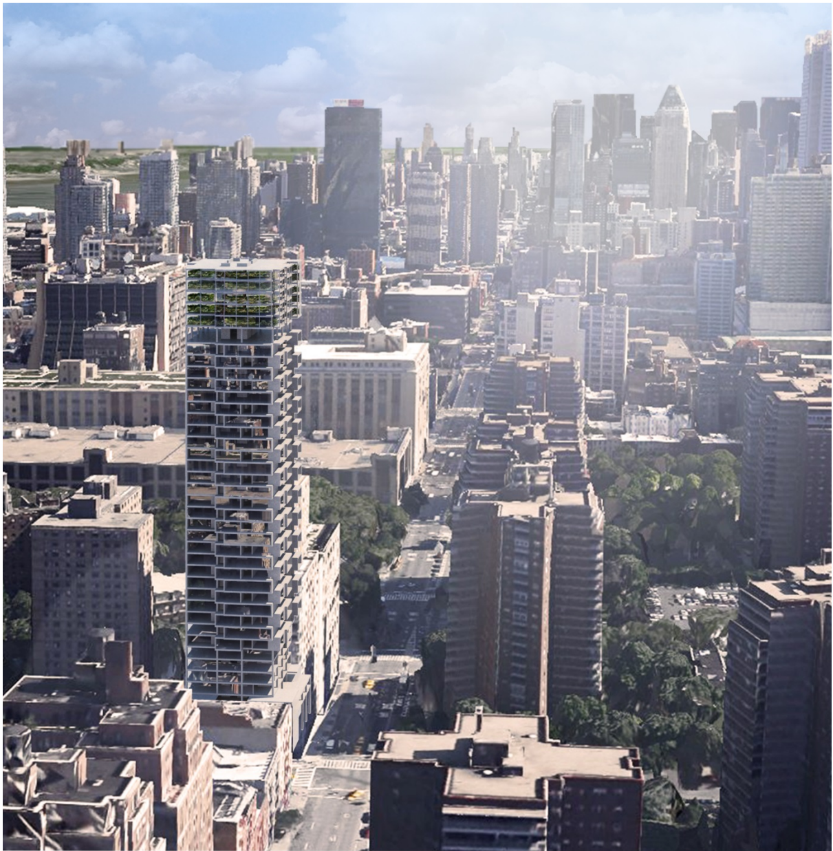
Figure 53.3 General view of Kilometro Zero Tower
