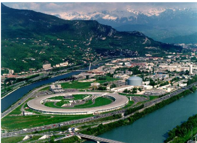
Figure A.1: Aerial view of the European Synchrotron Radiation Facility (ESRF), Grenoble (FR) [22].
