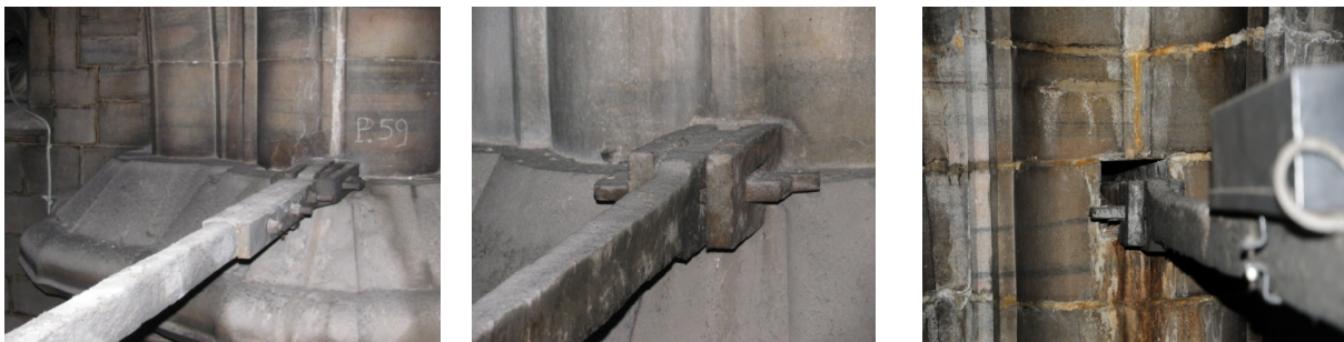
Figure 17: Clamping of the ties in the columns
