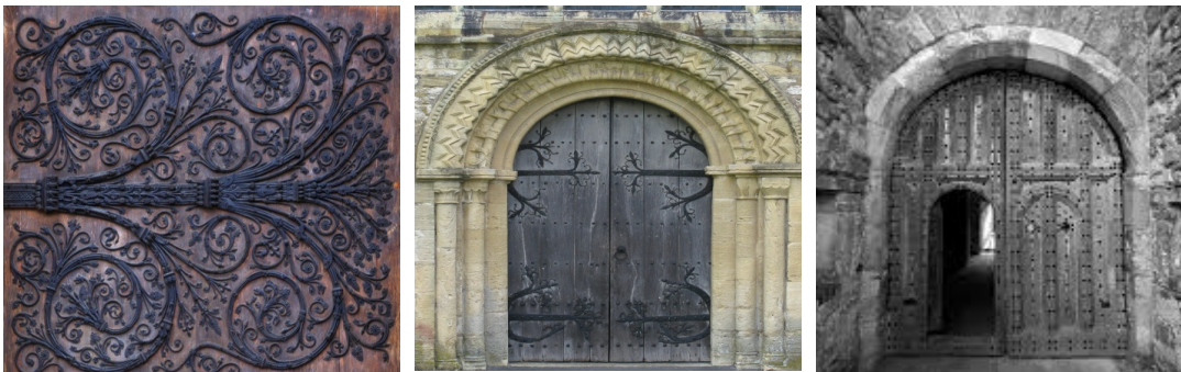
Figure 8: From left to right: West portal of Notre Dame de Paris; Split-curl hinges at St John the Baptist, Burford, Oxfordshire; The entrance to the gatehouse at Upnor Castle in Kent
