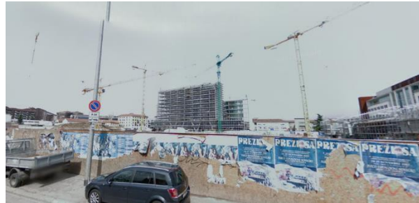
Cell id: 6858 Via Carlo Imbonati – construction site to commercial and residential
