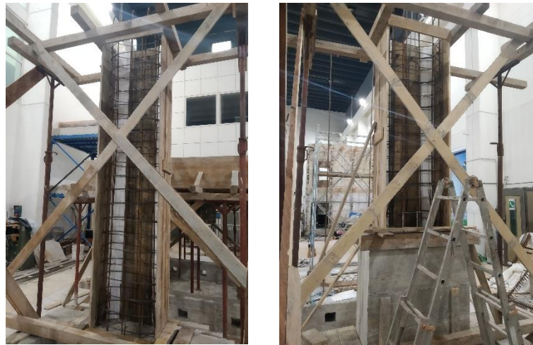
Figure 119: Pier shaft reinforcement pattern
