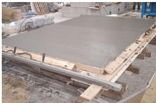
Figure 122 : Concrete casting of the slab
