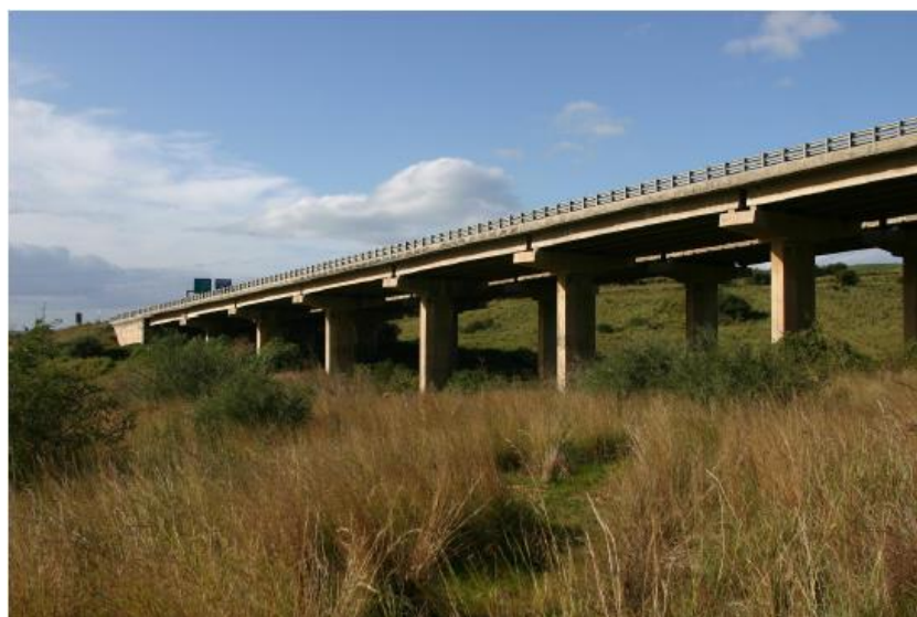
Figure 105: Global side view of the two Sordo Viaduct roadways
