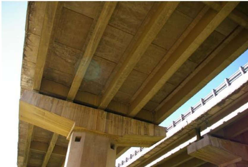
Figure 107 : Bottom view of the two viaduct roadway
