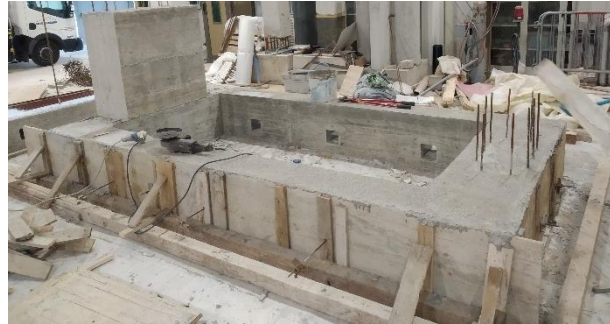
Figure 118: Foundation beam and pier basement
