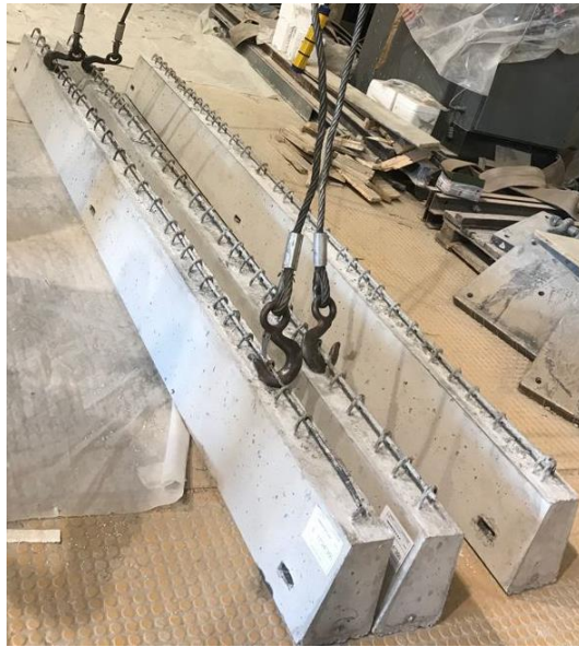
Figure 121 : Prefabricated prestressed deck beams
