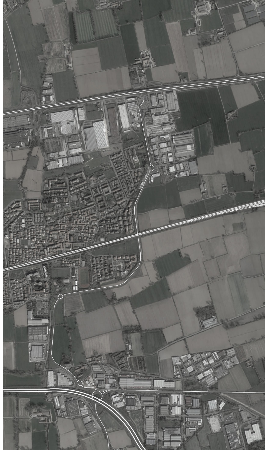
Figure 37. Milano-Melzo Terminal 2020. Figure by Author, Google Earth.
