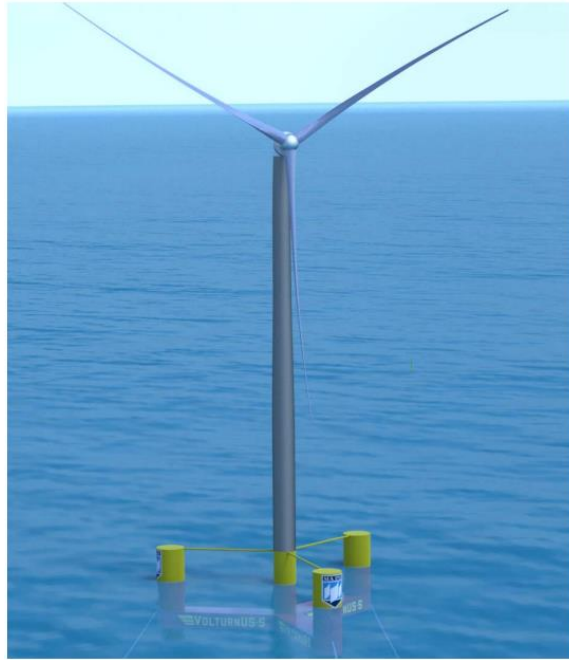
Figure 1.1: Rendering of the IEA 15-MW Offshore Reference Wind Turbine with UMaine VoluturnUS-S Reference Platform. Figure courtesy of the University of Maine.
