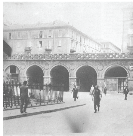
stone rail viaduct, 1880s
