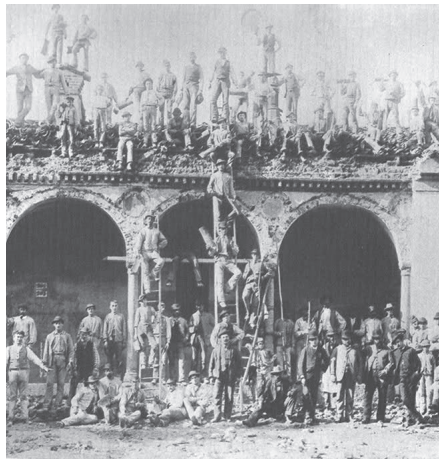
Lazzaretto, during demolition
