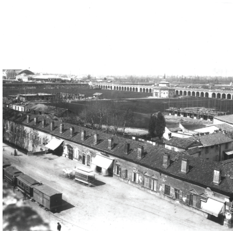
rail viaduct across the Lazzaretto, 1880
